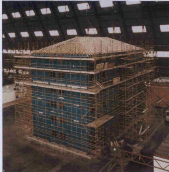
Figure 7-15: Timber frame construction tests Source: (Palmer and Heriot, 1999)
