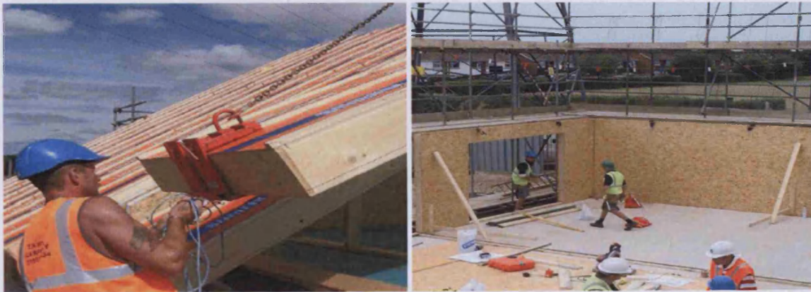
Figure 7-3: Panel system (timber frame) Source: (Hague, 2006)
