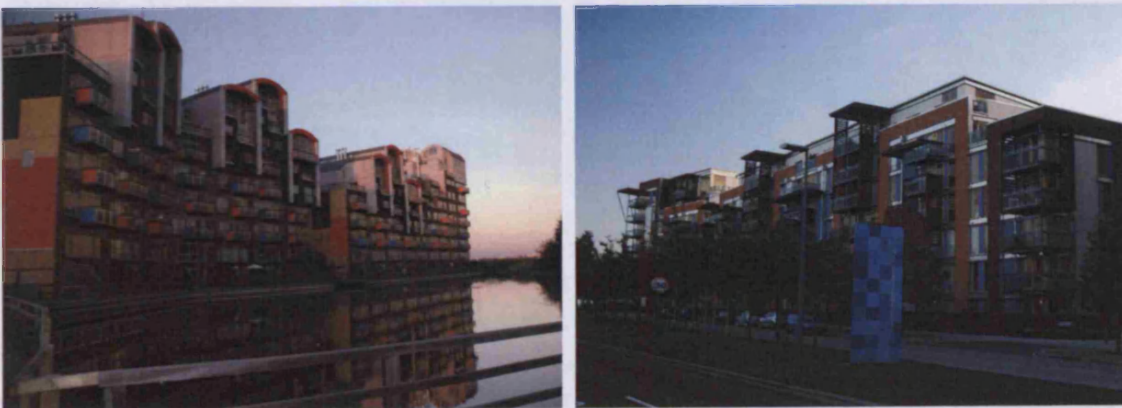
Figure 7-11: Some views of Greenwich Millennium Village Source: The Author
