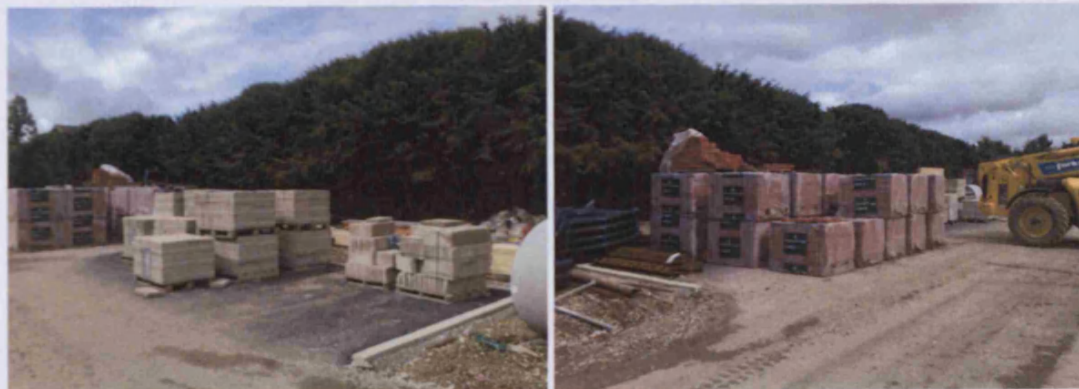
Figure 8-12: Construction material storage on site (UK) Source: the author
