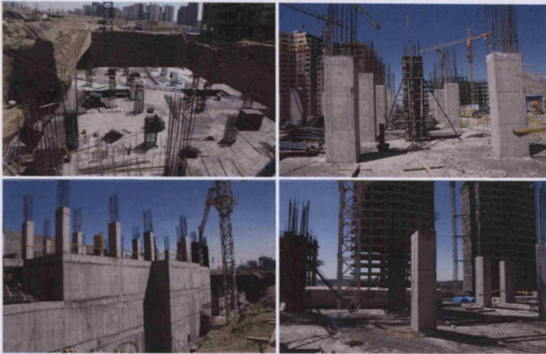
Figure 8-6: Construction methods in Tehran (RC frame)
