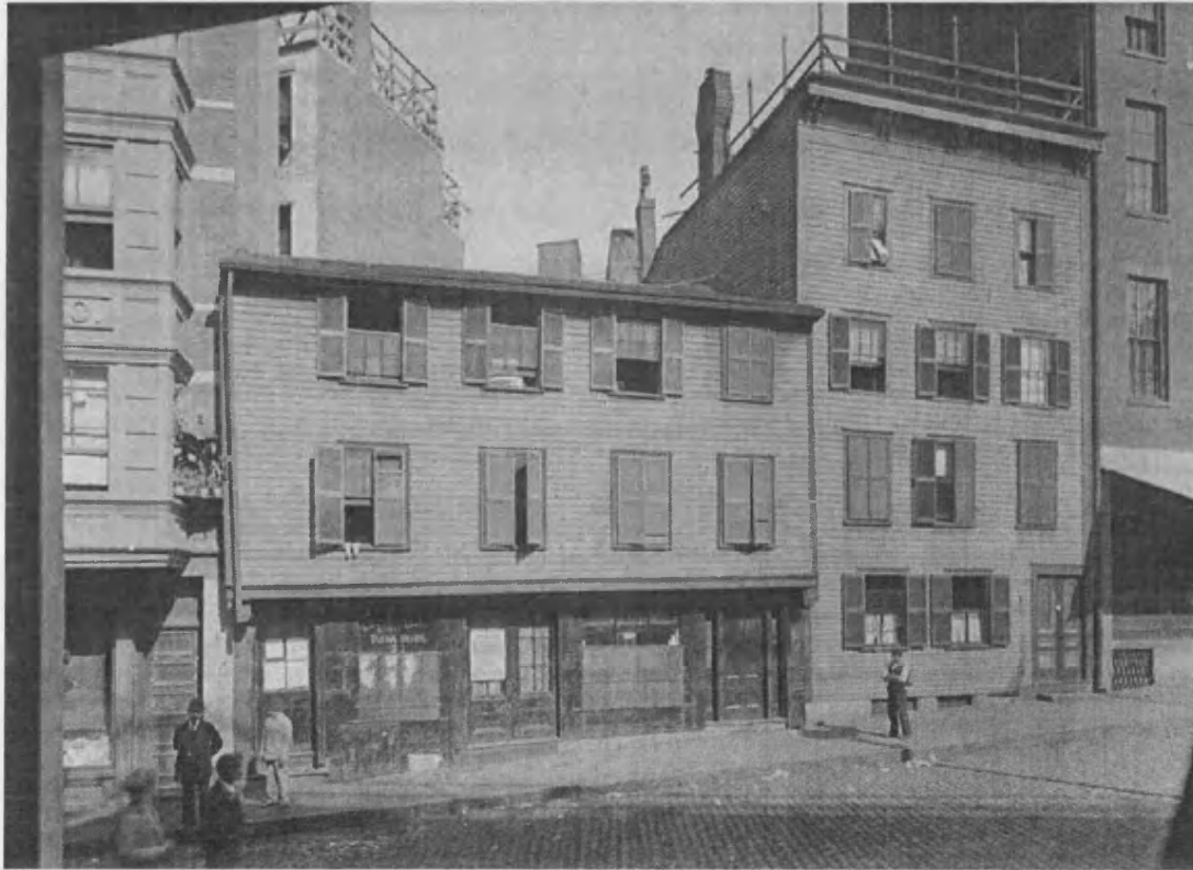
4-3. Revere House (centre-left) before restoration /NYPL
