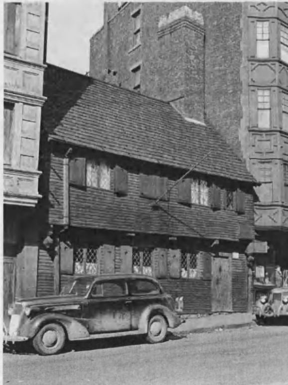
4-4. Revere House restored, 1930s /LOC
