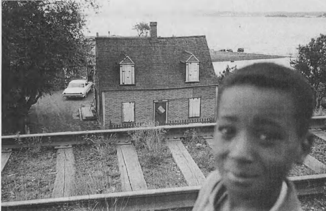
6.4-7. Ralph Jones House, prior to demolition, c. 1965 (Brooks) /NSARM
