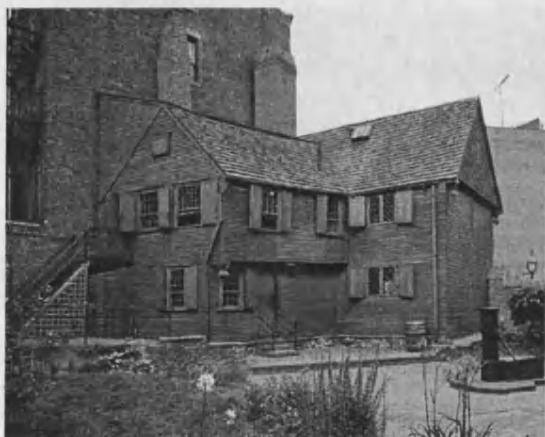
4-5. Revere House, rear elevations /LOC
