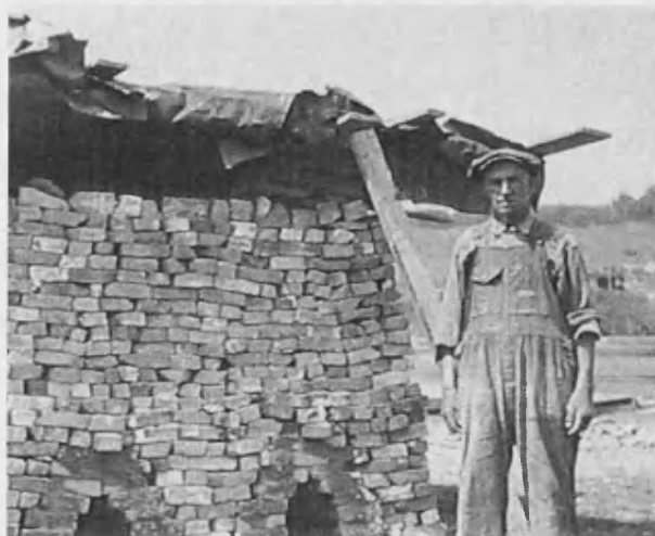
6.1-6. Making bricks on site for the Habitation reconstruction, 1939 /AHS
