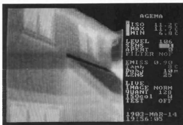
Figure 112: Thermography Survey - North Façade
