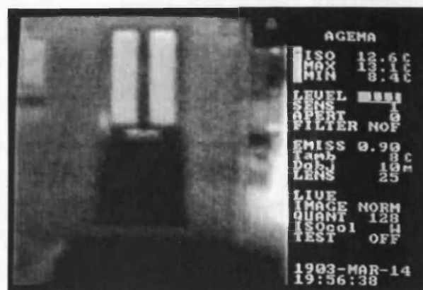
Figure 113: Thermography Survey - Front Door
