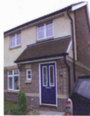
Figure 41: Typical contemporary house (Wimpey Homes, volume housing)
