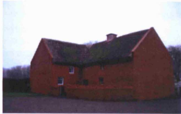
Figure 31: Traditional Stone Cottage with Lime Render (Source: National Museum of Wales)
