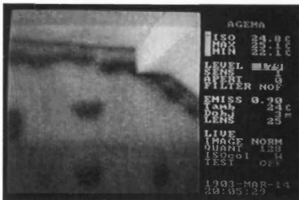
Figure 114: Thermography Survey – Dining Room West Wall
