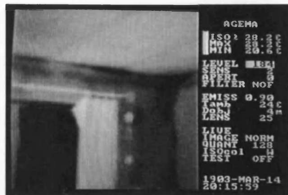
Figure 115: Thermography Survey – Lounge – North Facing Wall and Party Wall
