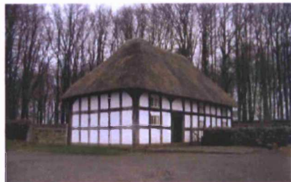
Figure 30: Traditional Timber Frame and Cob House (Source: National Museum of Wales)
