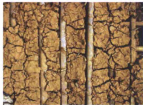
Figure 32: Typical Cob Wall Construction – Vulnerable to Driving Rain
