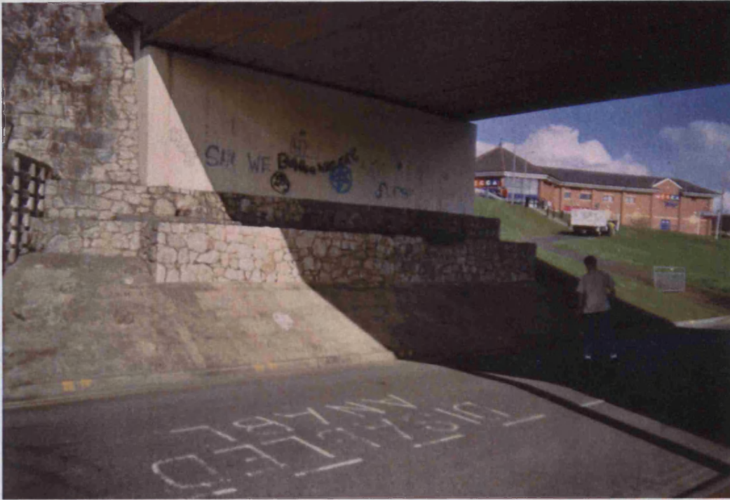
Photograph 6.8 Under the flyover – Photographer: Declan
