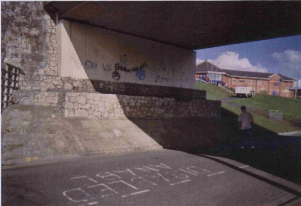
Photograph 7.6 Under the flyover – Photographer: Declan
