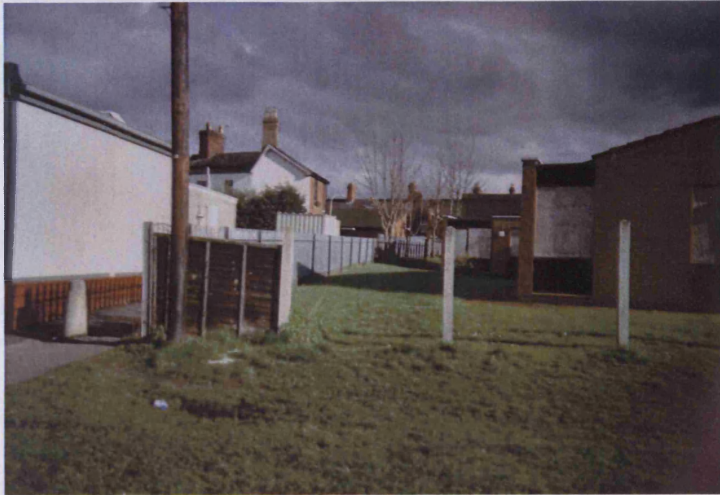
Photograph 7.4 Boarded up building – Photographer: Oli
