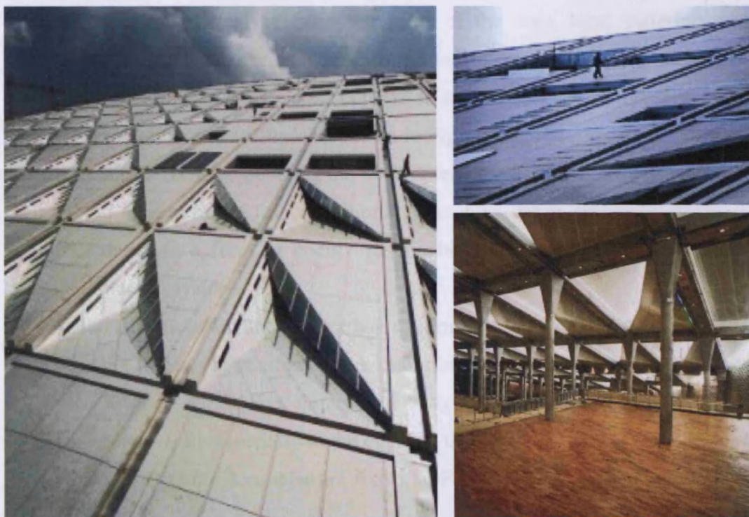
Figure 3- 24: The roof glazing and cladding from outside to notice its huge size, and from inside to notice the light distribution. (Source: TLA, 2006)
