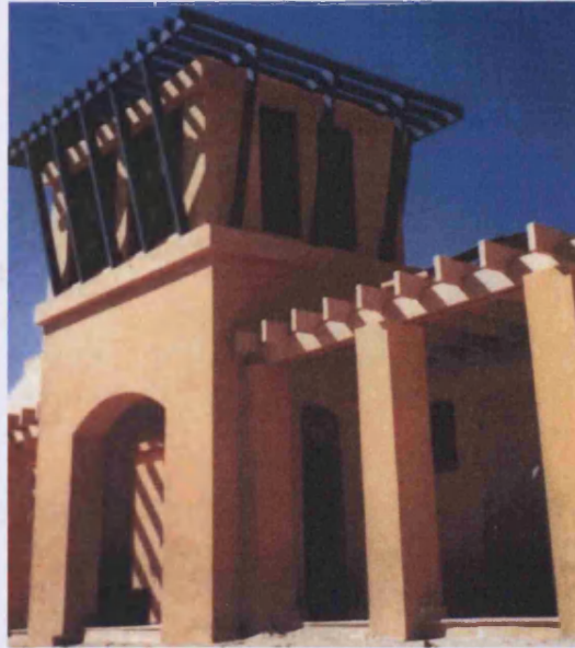
Figure 3- 18: Modern style ventilation towers, maximize air movement in outdoor corridors. (Source: El Gouna, 2009)
