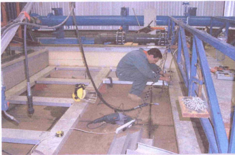
Figure 5.4: Strengthening of basin foundation
