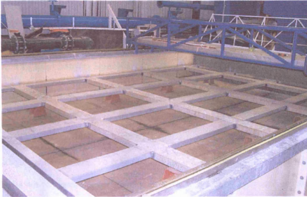
Figure 5.5: New basin floor base structure
