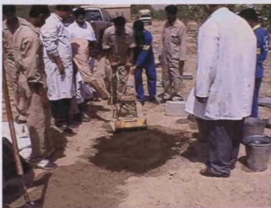
Plate 8.3. Backfilling and compacting the test beds
