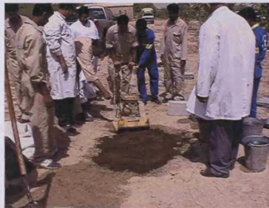
Plate 8.2. Mixing the Sabkha soil with oil residue
