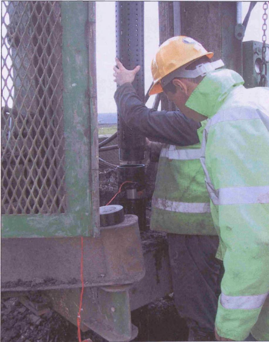
Figure 6.5: *A photograph illustrating attachment of an electrode array onto the exterior casing surface during emplacement of a gas recovery well at Nantygwyddon (Jeremy Jones, Encia Consulting Ltd).*
