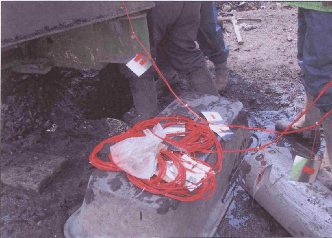
Figure 6.4: A photograph illustrating a pre-fabricated electrode array comprising single-core electrical cables and stainless steel sheet electrodes prior to emplacement within the landfill (Jeremy Jones, Encia Consulting Ltd).
