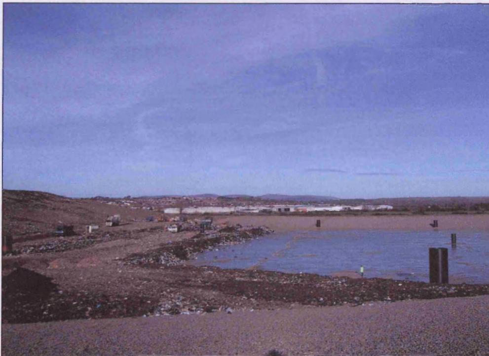
Figure 5.9: *A photograph illustrating progressive burial of the electrode array by a series of refuse raises (author).*
