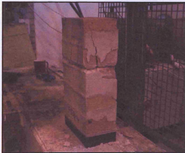
Plate 7.2- Typical failure pattern in prototype tests.
