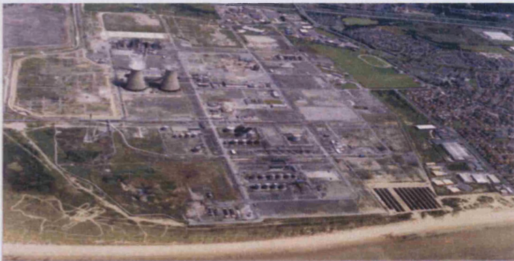
Figure 3.4 Petrochemical factory in 2000 after many of the plants had been decommissioned and demolished
