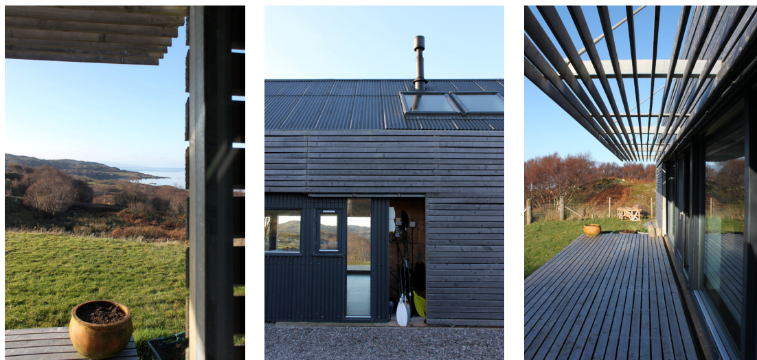
Fig. 7.27 Interrelationship between landscape and dwelling at The Shed; Fig. 7.28 Form has shutters to provide protection from the weather and for storage; Fig. 7.29 Form is responsive to site and climate with external solar shading
