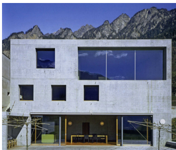
Fig. 7.116 Simple monolithic elevation of House in Chur using cast in-situ concrete
