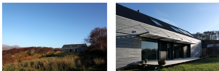
Fig. 7.30 The Shed, Tokavaig, Isle of Skye is sited to make best use of landscape and views; Fig. 7.31 It is highly insulated and economically clad in corrugated fibre cement and larch, with sliding shutters to protect from storms
