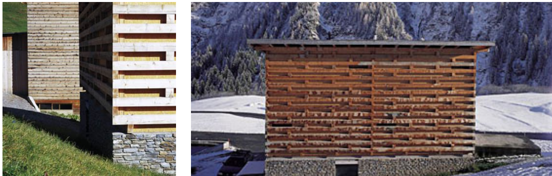
Fig. 2.13 The slaughterhouse by Gion A. Caminada - a stone platform with a timber structure above; Fig. 2.14. Uses traditional, local materials
