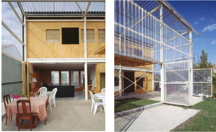
Fig. 2.15 Latapie House, Floirac by Lacaton and Vassal is low budget and fits into the street profile of a discontinuous residential area of Bordeaux's inner suburbs; Fig. 2.16 Materials used are polycarbonate and timber shuttering
