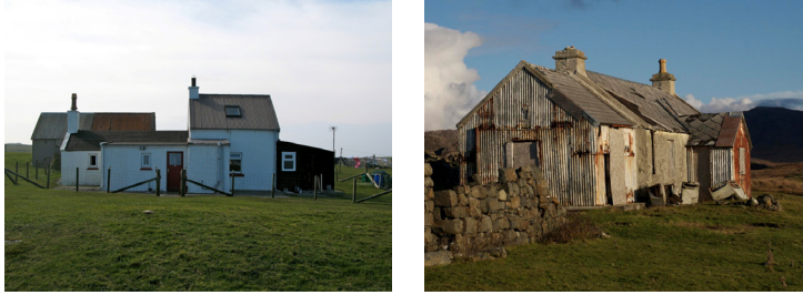
Fig. 7.37 Ad hoc additions and outhouses influence the architecture of Rural Design; Fig. 7.38 House built from whatever resources available
