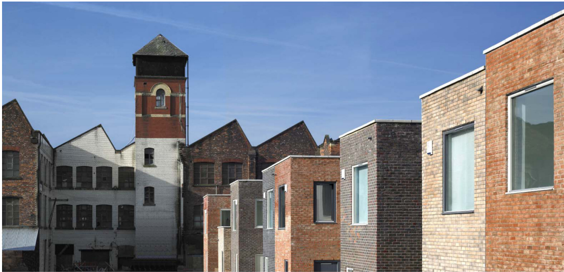
Fig. 6.34 Flat roofs contrast with the pitched roofs of the nearby mill building, whereas materials specified are similar in appearance
