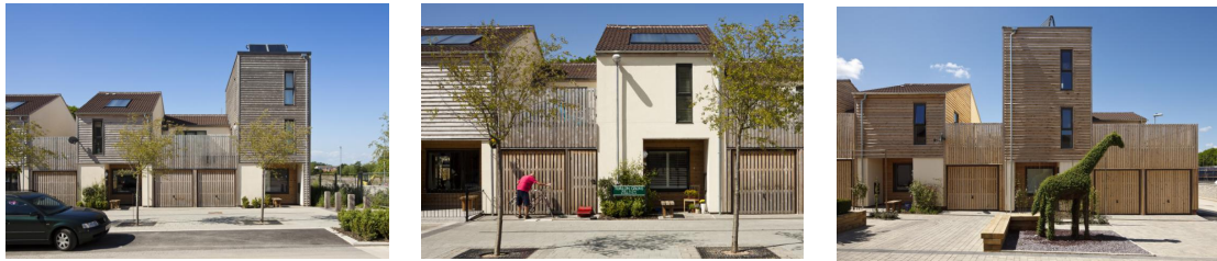
Fig. 6.30 Cedar cladding articulated to correspond with varying terrace form; Fig. 6.31 Elements are rendered; Fig.6.32 Roof terraces situated above the garages
