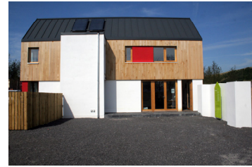
Fig. 4.41 South elevation: standing seam metal roof, timber cladding, Welsh sweet chestnut windows and doors, external insulated render system
