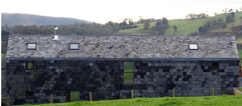
Fig. 4.37 Slate cladding on north elevation
