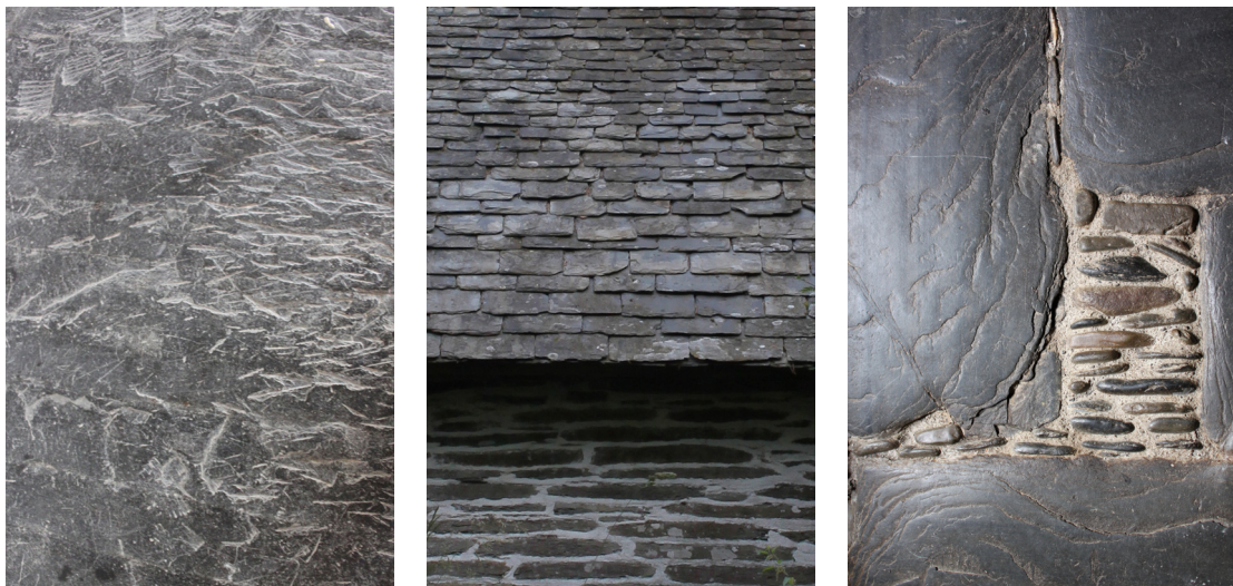
Fig. 8.13 Material textures and aesthetic quality created through construction and building use, Worktop showing marks of use; Fig. 8.14 Horizontal aesthetic created, materials in the construction get smaller towards the top; Fig. 8.15 Combination of large and small stones are use to make the flooring with the smaller stones used to fill in the gaps.
