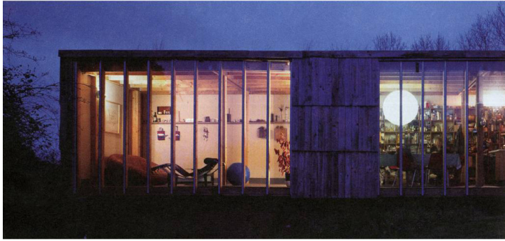
Fig. 4.50 Low tech house using passive principles – large area of glazing on the south façade
