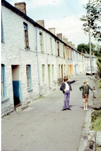
Fig. 6.16 Photograph showing different coloured window and door surrounds at the Triangle, Pentrebach, taken in 1972
