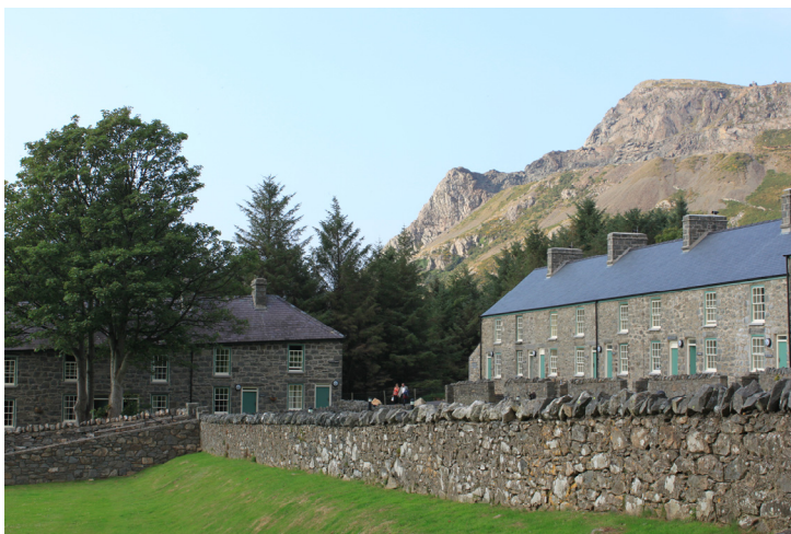
Fig. 6.8 Materials used to build Nant Gwrtheyrn quarried from the mountainside in a remote and inaccessible part of the Llyn Peninsula
