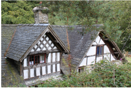
Fig. 4.25 Gilfach longhouse with an elaborate elevation to the roadside to show off wealth
