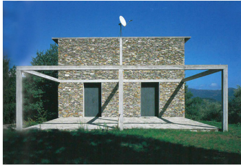
Fig. 7.120 Casa de Piedra at Tavole by Herzog & de Meuron; Fig. 7.121 Detail of wall construction - concrete structure with dry stone wall infill
