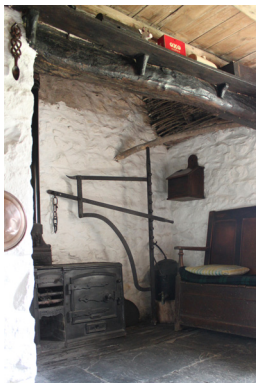
Fig. 7.11 Inglenook fireplace at Bryn Eglur with wicker fireplace hood
