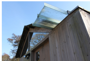
Fig. 7.42 Simple form and detailing of materials at the pottery in Cheriton in the Gower; Fig. 7.43 U shaped glass cladding sections used as roof lights to exhibition space and gutters
