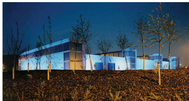
Figure 32 Gateway factory at Baglan Energy Park
