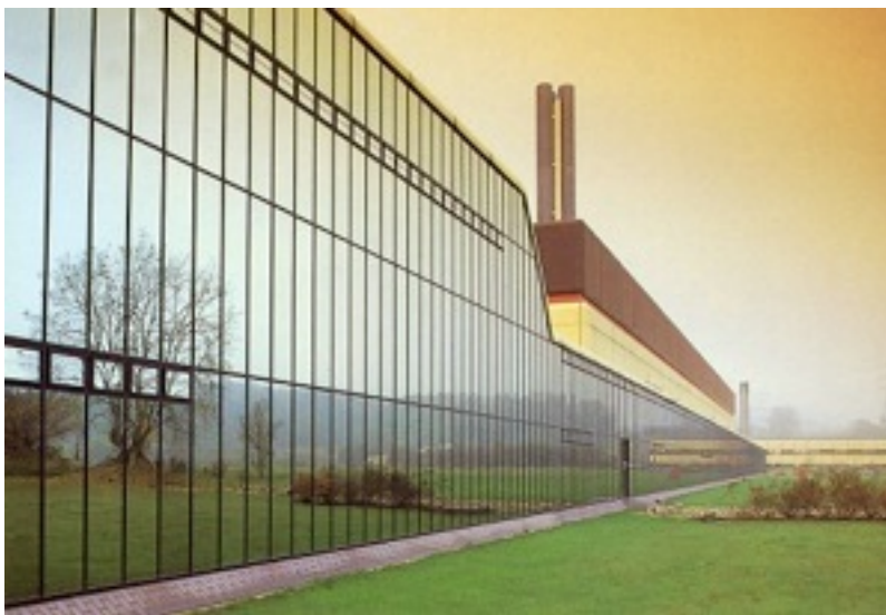
See Figure 4.8. Amersham International Radiochemical Factory.
