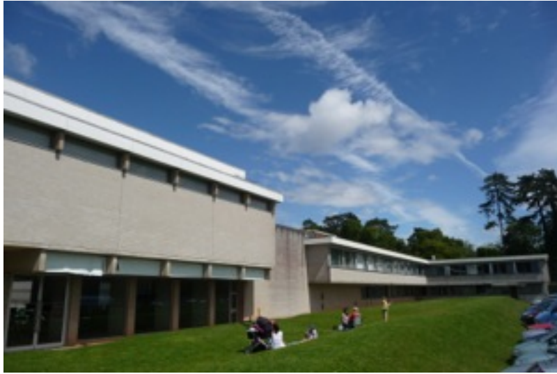
See Figure 6.12. South Elevation from the south west.
