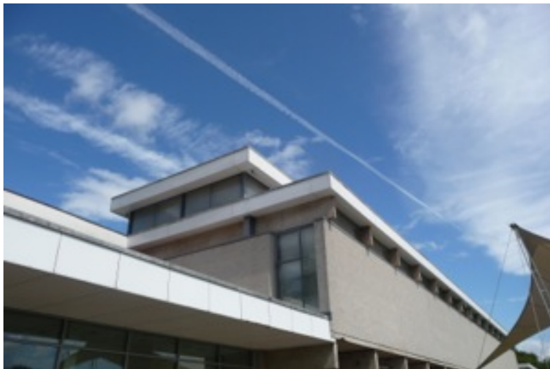
See Figure 6.16. Detail showing the conjunction of the restaurant block with the Agricultural Gallery and ‘lantern’ storey over.
