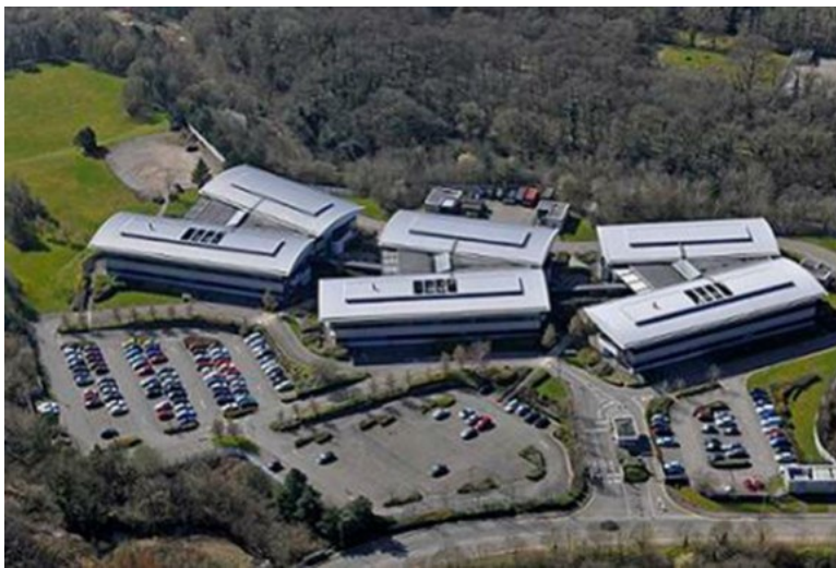
See Figure 4.9. British Airways Avionics Facility.
