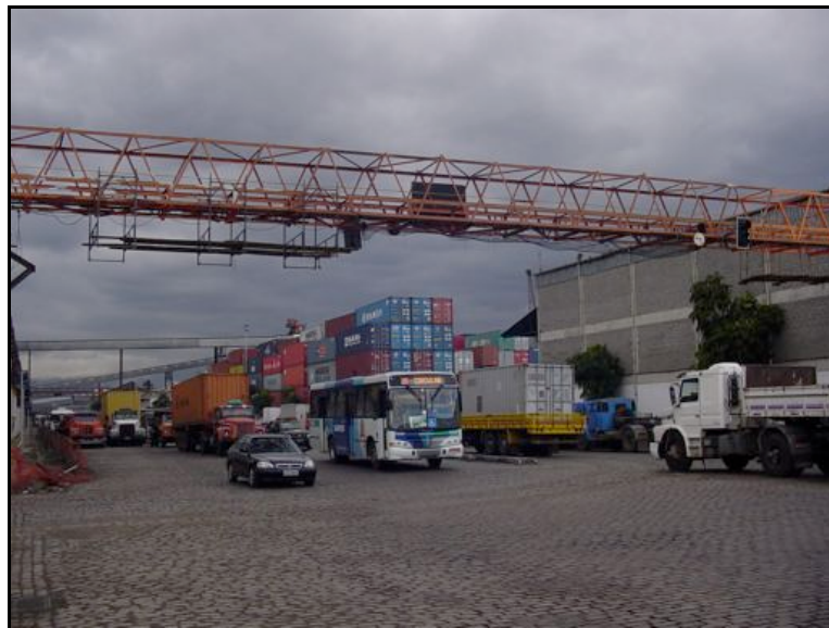
Figure 2.1: Busy port of Santos Source: Eliseo Lucero-Prisno III
