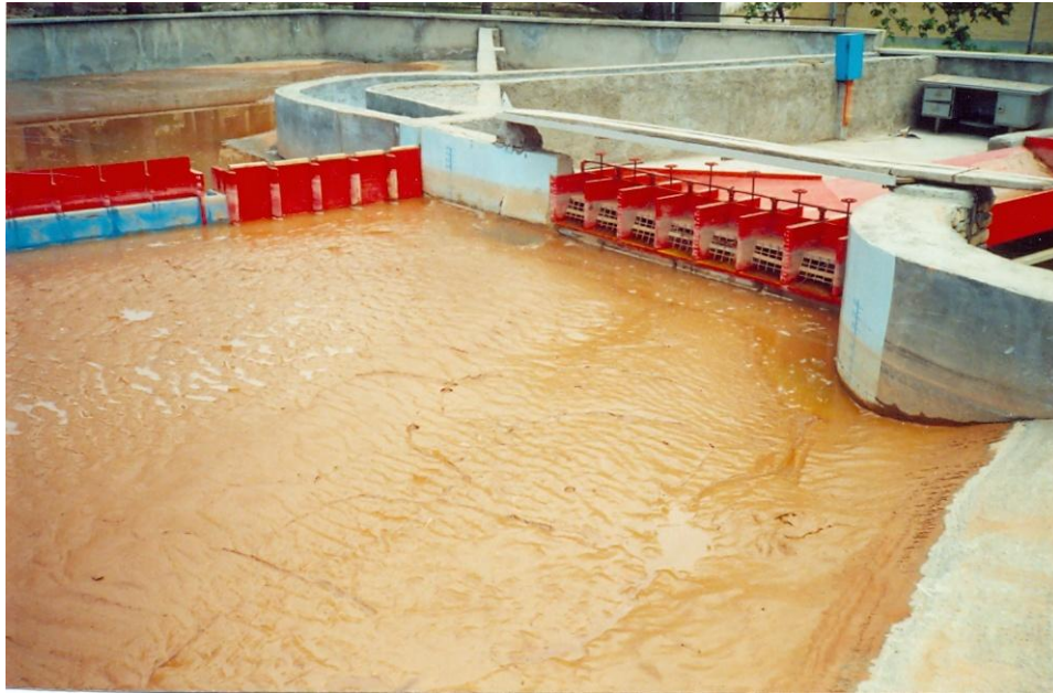
Figure 3.27 The dredging zone in front of Azadegan intake after tests
