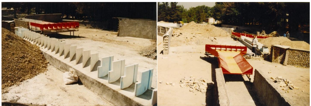
Figure 3.9 The installation stage of the physical model
