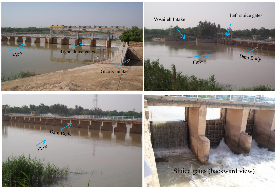
Figure 3.6 Pictures of existing hydraulic structures of Hamidieh regulated reservoir
