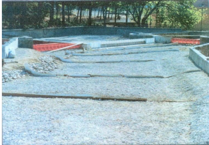
Figure 3.10 Constructing bed topography for the reservoir model
