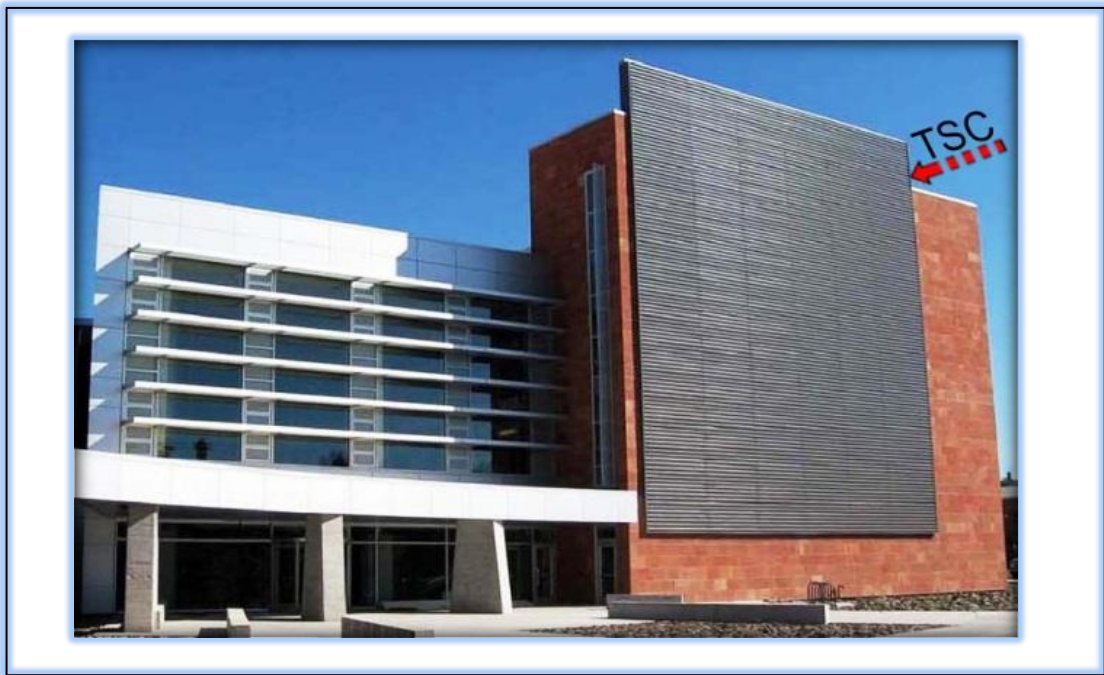
Figure 5-19: Façade integration – TSC (Ariz), Northern Arizona University Distance Learning Center, USA (CA Group 2011)
