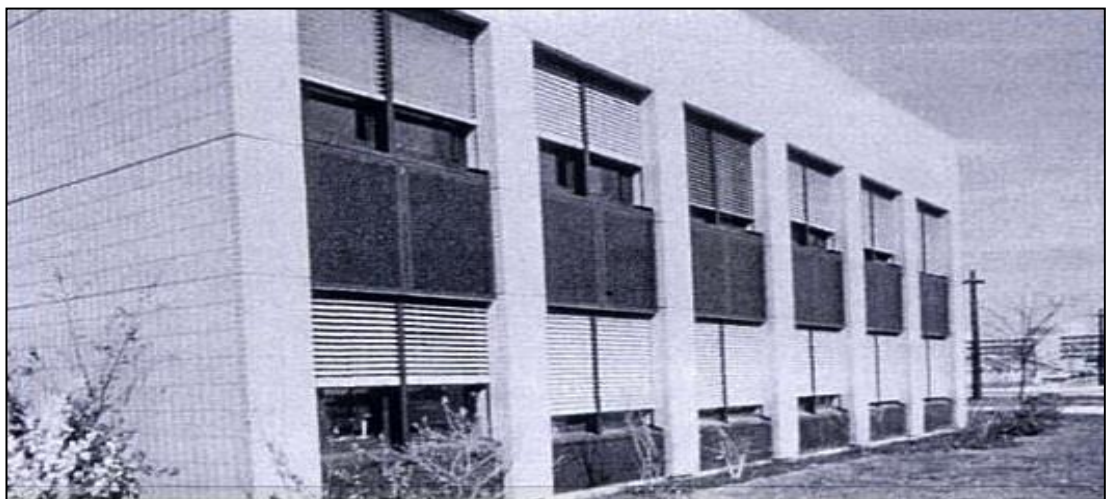
Figure 3-5: The LRE building at EPFL (École Polytechnique Fédérale de Lausanne) in Lausanne, Switzerland (Sick and Erge 1996)
