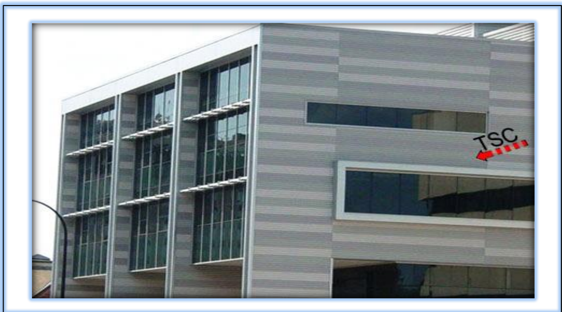
Figure 5-15: Façade integration of TSC (Ann), Ann Arbor Municipal Building, USA, InSpire wall (ATAS 2010)
