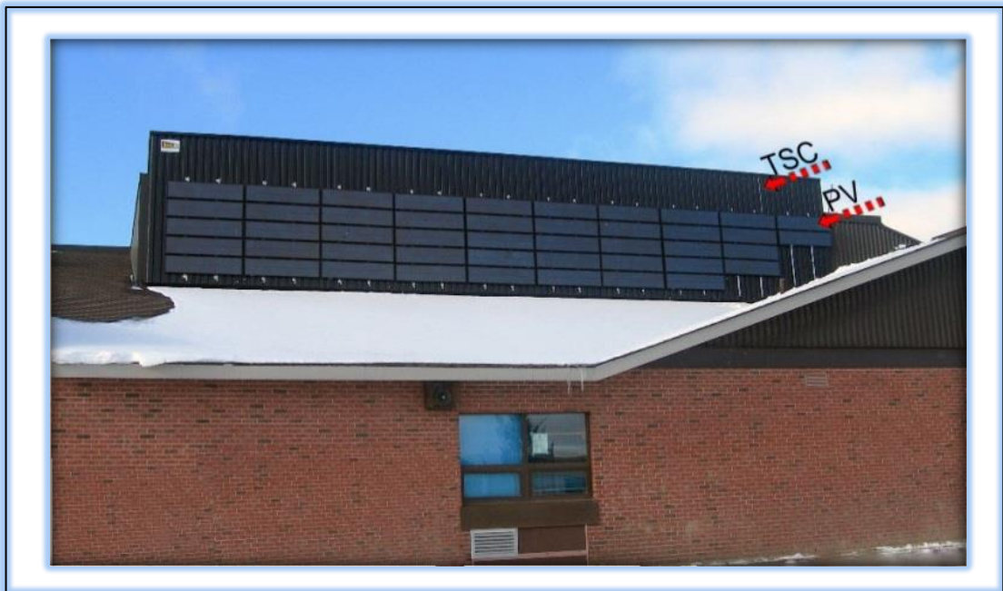
Figure 5-23: Façade integration – PV/TSC (Marg), St Marguerite Bourgeoys School, Ontario–Canada (SolarWall n.d.)
