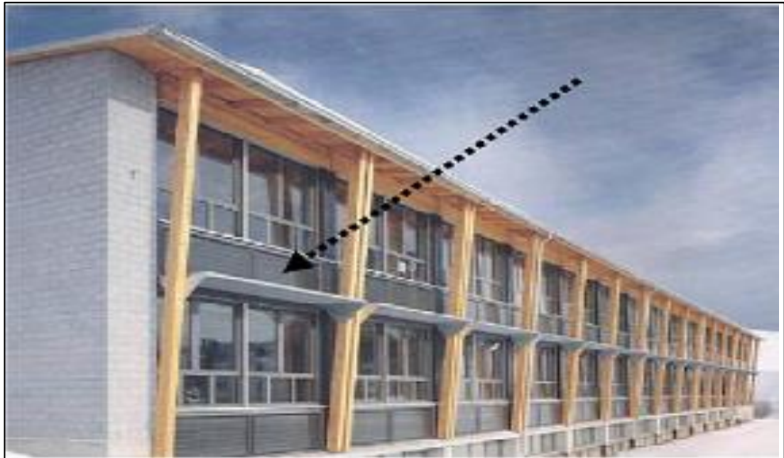
Figure 3-7: Glazed collector at Upperstage centre in Germany (Probst and Roecker 2007) as arrowed
