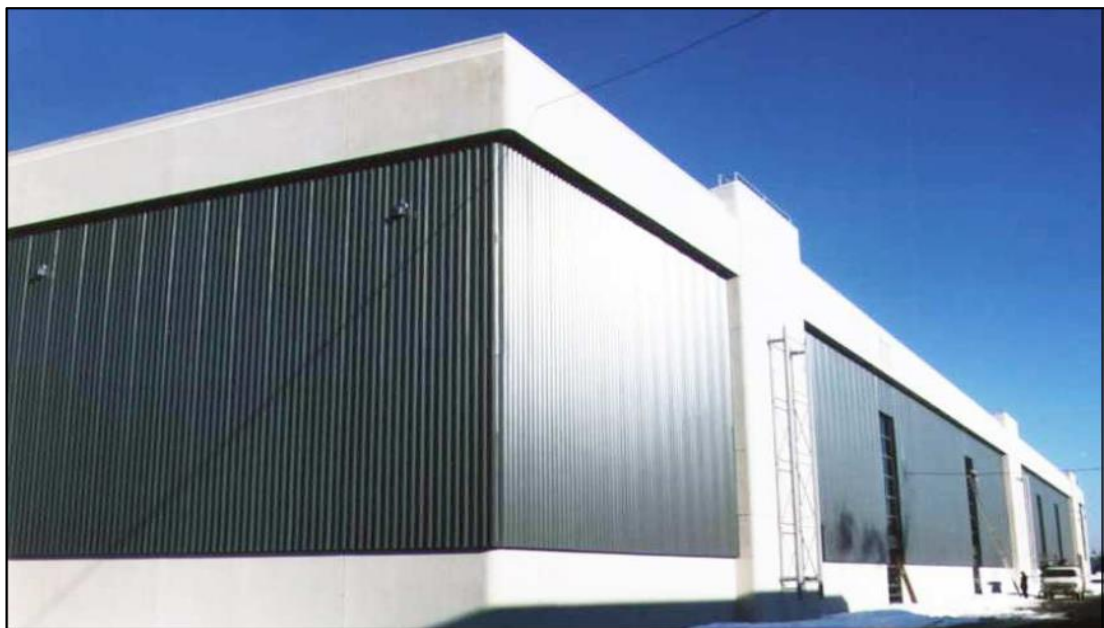
Figure 3-8: TSC industrial Canadair facility in Canada (SolarWall 1996)
