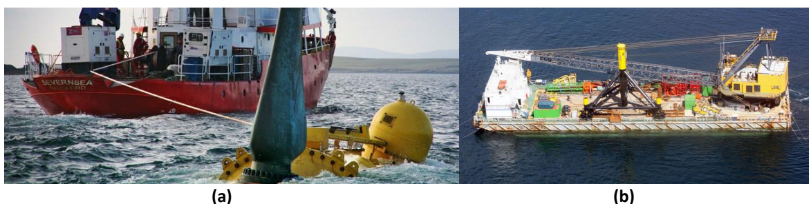
Figure 33 Tidal Generation Ltd turbine Installation (a) Nacelle (b) Foundations (Alstom, 2013)
