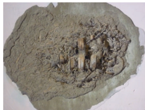
Figure 4: Detail of quincha wall build-up.
