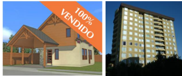
Figure 2: Condominio Frankfurt (100% sold) [24] Figure 3: Rotterdam building. Author's photo
