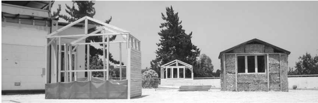
Fig. 5. Construction of physical test chambers, progress January 2010
