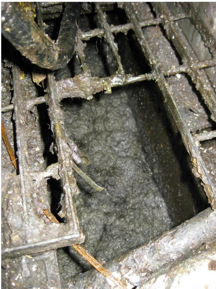
**Figure 13 Sludge within a Sump**
