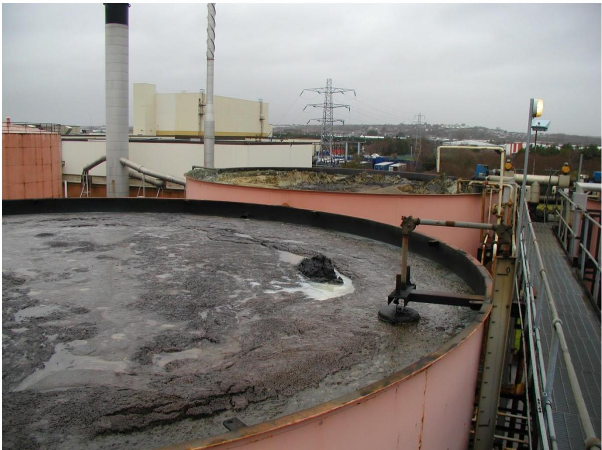
**Figure 16 Two Types of Sludge in the Wastewater Storage Tanks**
