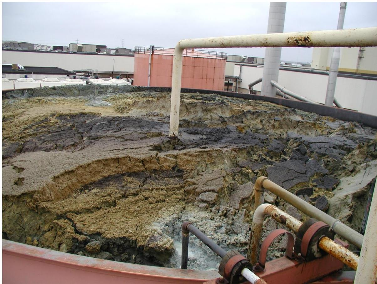
**Figure 18 Higher Viscosity Sludge in Tank 4**
