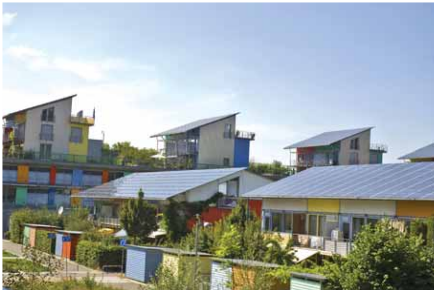
Solar Settlements with plus-energy houses - These houses are part of the “Solar Siedlung”, a 50 plus-energy building settlement of Vauban district in Freiburg, Germany. Over the year, these plus-energy houses produce more energy through renewable energy than they consume due to their low-energy construction design. The inhabitants of this district are particularly environmental conscious: every third resident has chosen to live car-free. © rsester/Fotolia
