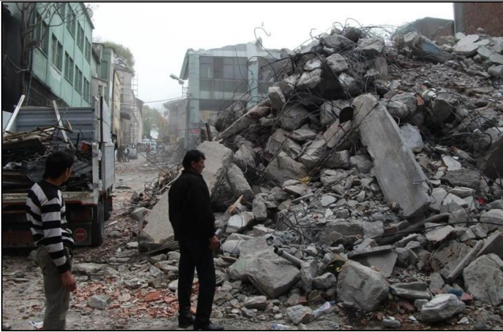
Photos from the demolition day, 17 th April 2012. (Source: Personal Archive)
