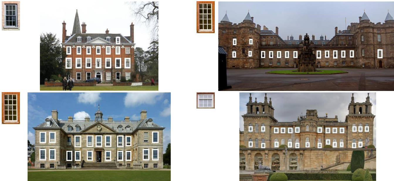
Fig. 3 HOG-based template matching over varying scales on Flickr images of UK heritage properties Welford Park 3 ( top-left ) and Holyrood Palace 4 ( top-right ), a Wikipedia image of Belton House 5 ( bottom-left ) and a Flickr image of Blenheim Palace 6 ( bottom-right ). For each image the template used is shown top-left, with matches as thick white bounding boxes .
