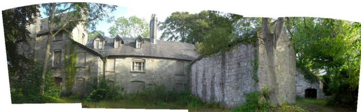
Figure 64: Western elevation of Plas Dulas illustrating the three main series of construction from right to left: late-eighteenth, early-nineteenth and mid-nineteenth century, 2009. Mark Baker.
