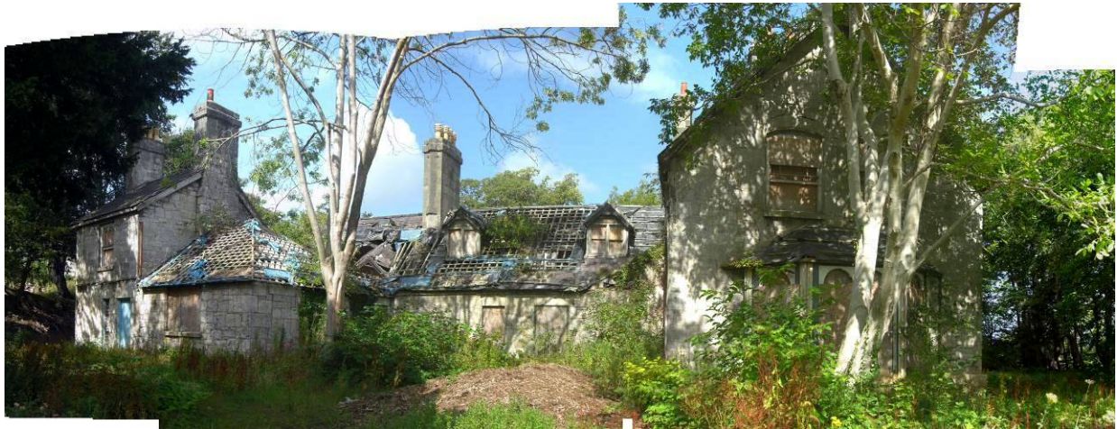
Figure 63: Eastern elevation of Plas Dulas, showing the early nineteenth century farmhouse on the left-hand side, with the farmhouse extension in the centre and the mid-nineteenth century villa on the right-hand side, 2009. Mark Baker.
