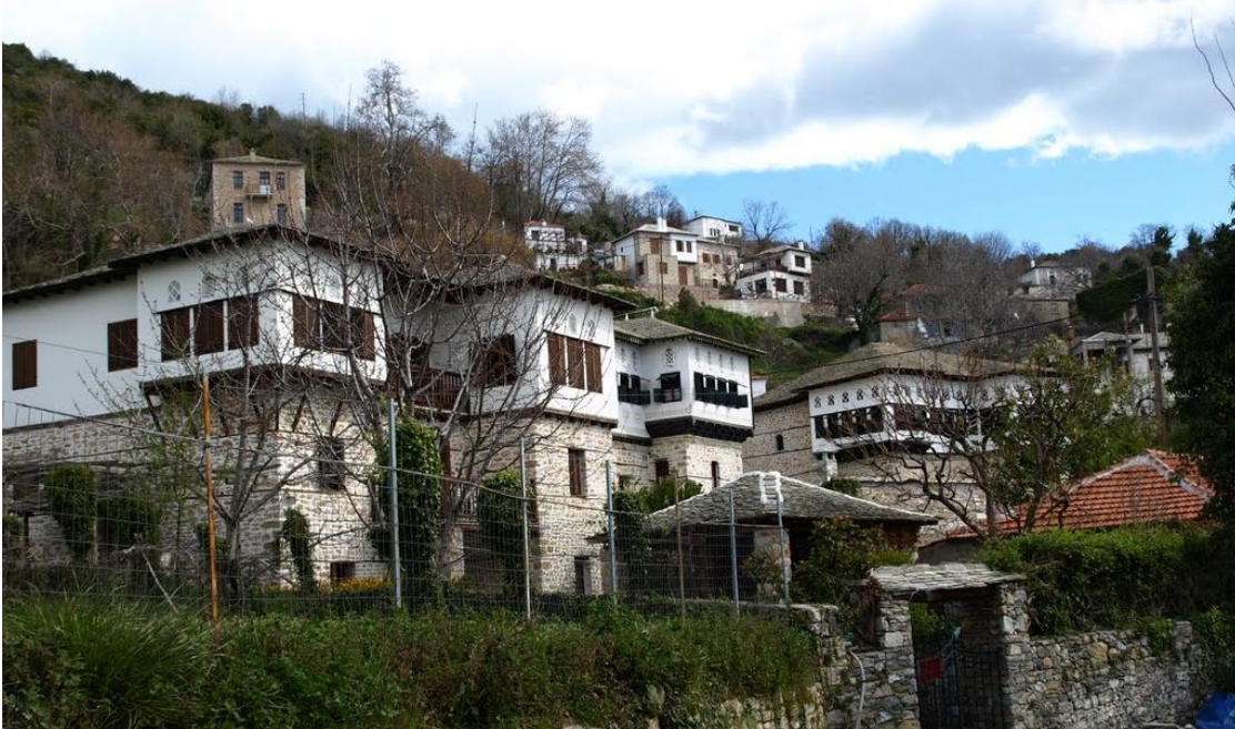
Figure 3: Built environment in Vizitsa
