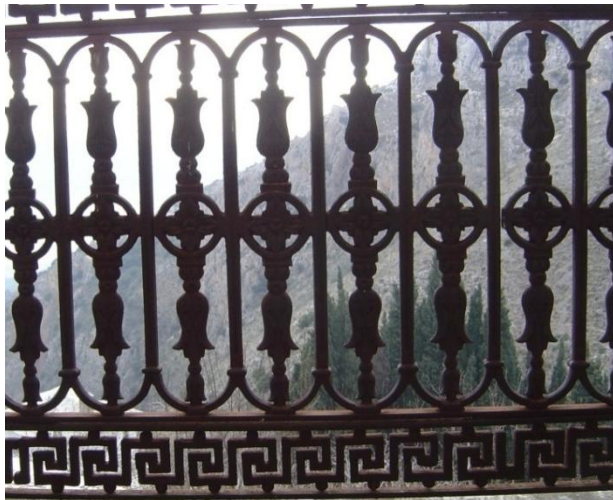
Figure 41: Balcony metallic details
