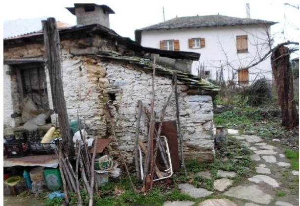
Figure 53: Built oven in Mouresi
