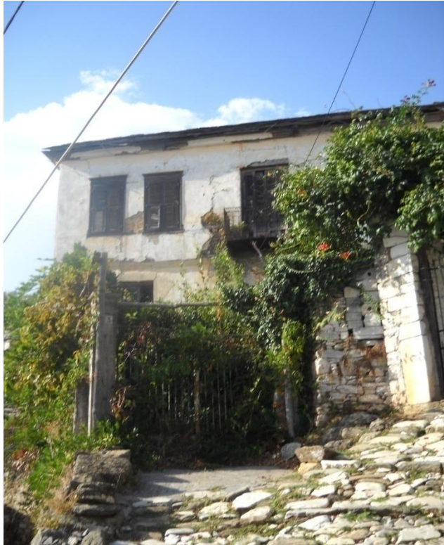
Figure 64: Derelict mansion house in Agios Lavrentios
