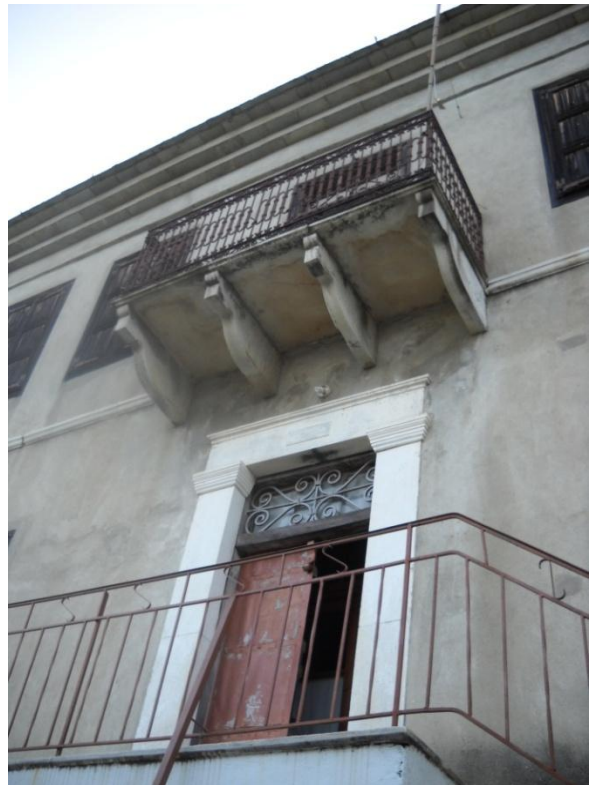
Figure 44: Marble detail in the balcony
