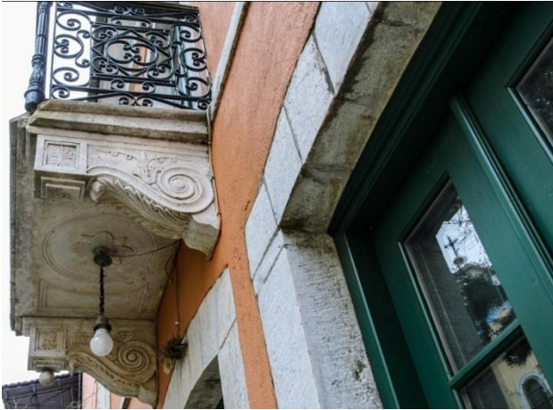
Figure 5: Details in the balcony
