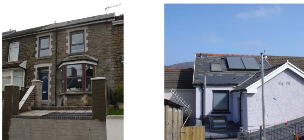
Figure 4.21: Dwelling 5, triple glazing windows and solar hot water collectors on the roof
