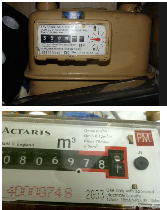
Figure 3.3: existing gas meter with dial(left) and reflective digit(right)
