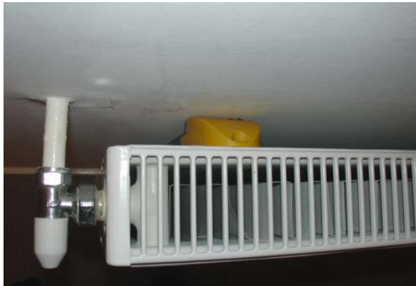
Figure 3.10: Radiator surface temperature monitoring as viewed from above.
