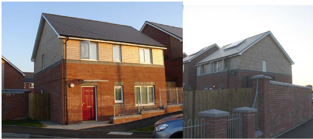
Figure 4.47: front and rear view of dwelling 8
