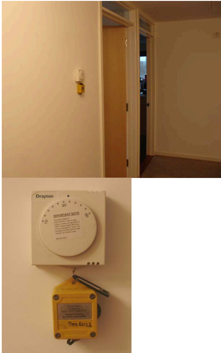
Figure 4.37: Thermostat in the hallway and electrical resistance logger
