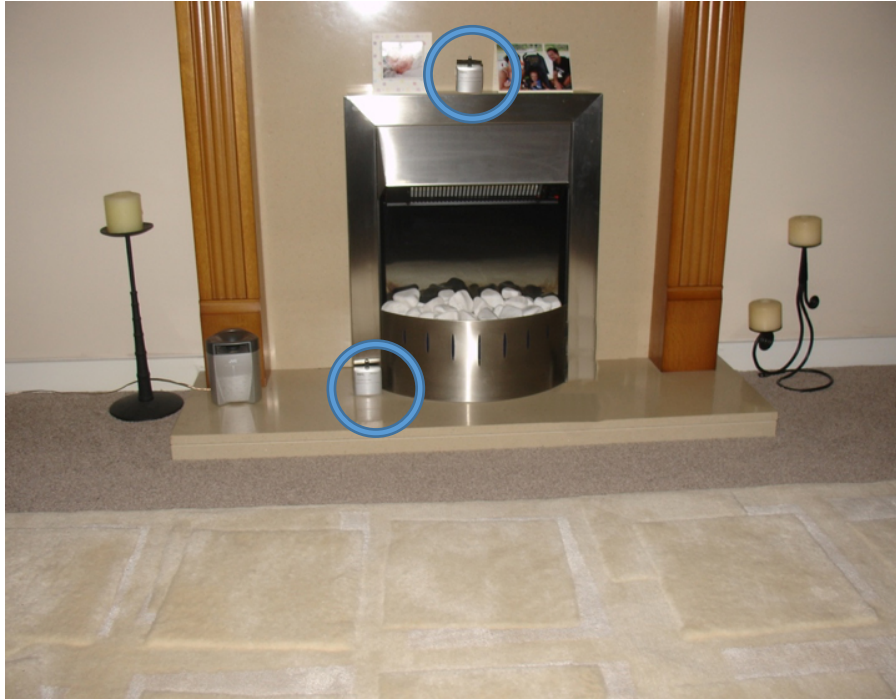
Figure 4.45: Wireless CO 2 sensor
