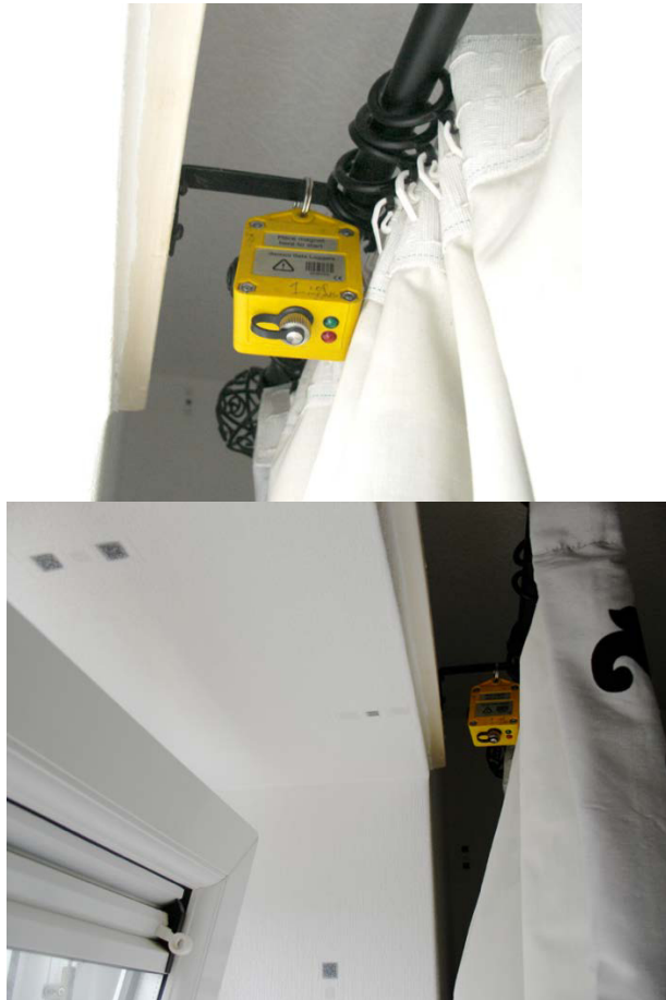
Figure 4.25: Additional temperature next to tilt-open windows
