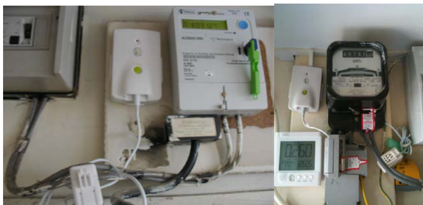
Figure 4.27: Owl current transducer on prepay electricity in dwelling 4 (left) and dwelling 5 (right)
