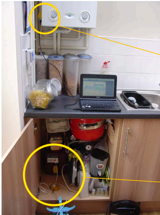
Figure 4.24: gas sub-meter installation with boiler in dwelling 5
