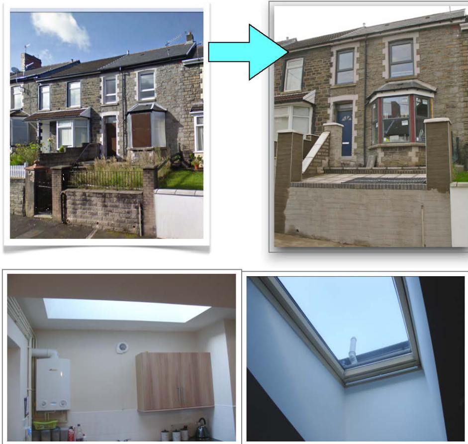
Figure 4.20: Fabric upgrade and skylight in the kitchen of Dwelling 5
