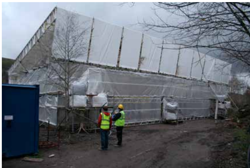
Fig 9.101 Enclosed scaffolding tent over construction site
