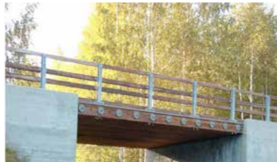
BELOW Fig 7.9 Stress laminated bridge slabs made up of glulam beams on Mattisdammen (top) and Daleråsen bridges (bottom), Norway
