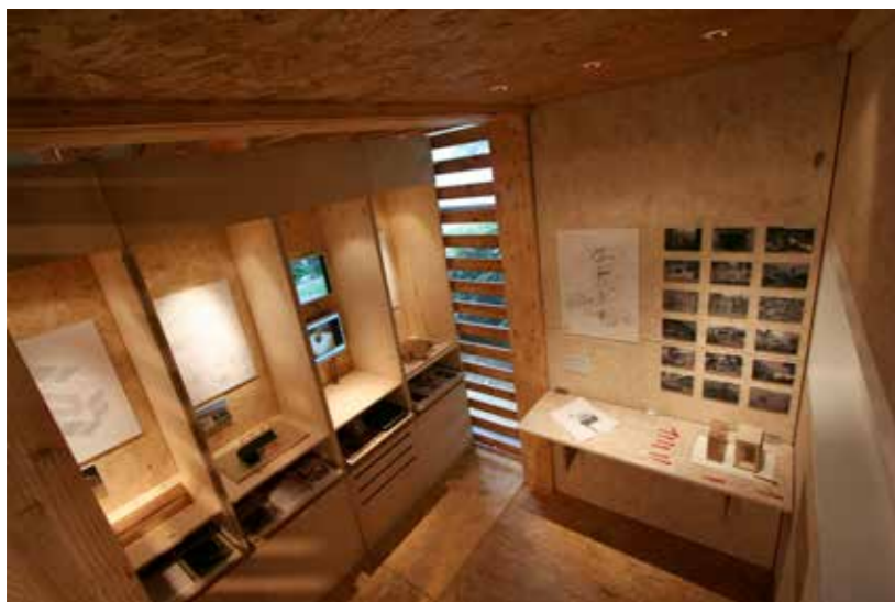
RIGHT Fig 10.11 600mm layout grid coordinated with the following: a. 150 x 150 x 1200mm frame b. standardised glulam post and beam structure c. timber frame panel d. 1200 x 600m plywood cabinets e. solid timber panels f. volumetric spatial arrangement and construction
