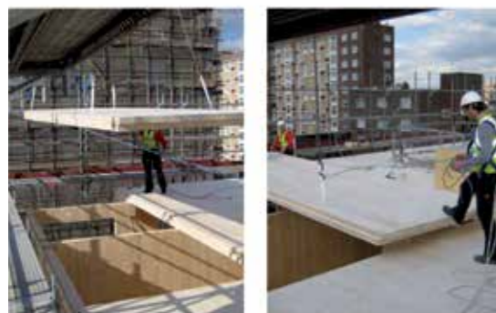
LEFT Fig 7.6 Site construction sequence: wall and floor panels
