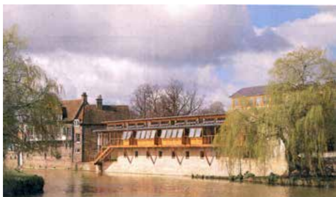
ABOVE Fig 6.14 Section through cantilevered study bay Fig 6.15 Detail of double beam bolts LEFT Fig 6.16 Green oak posts and double beam structure Fig 6.17 Oak clad exterior to river
