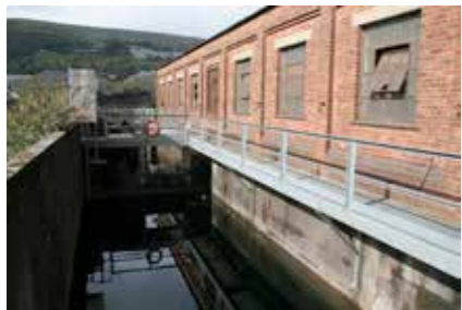
LEFT Fig 9.54 Existing photos of pumphouse and surrounding site
