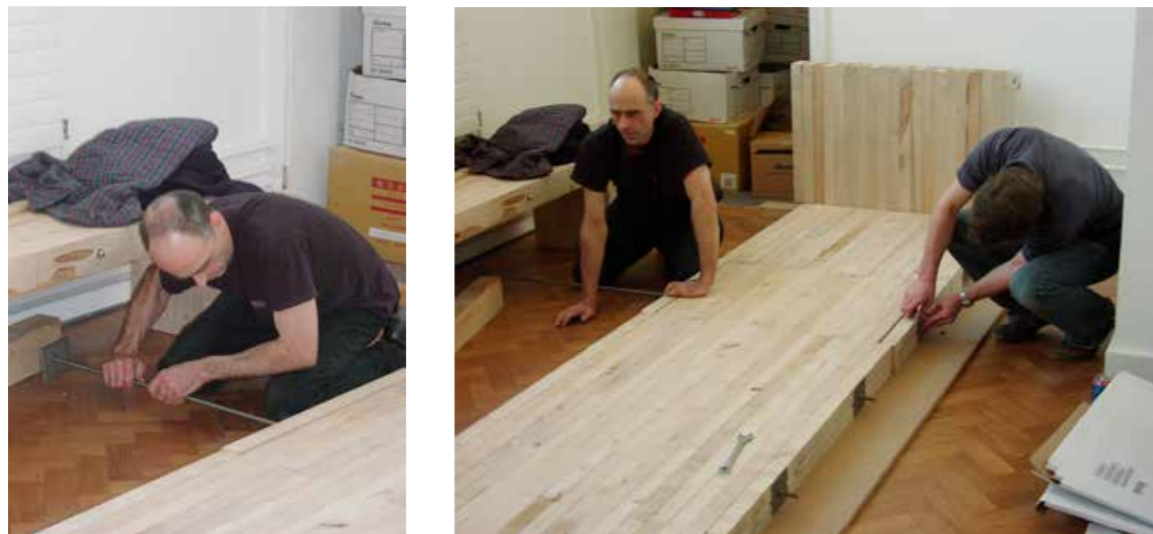
Fig 7.66 Installation sequence photos in Bute building
