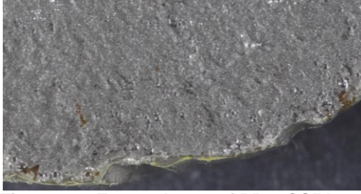
Figure 192 Zoomed area of PB72CS5A showing the corrosion formed and the gloss of the coating
