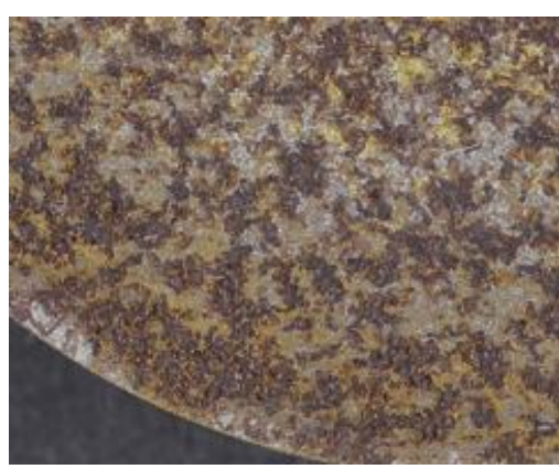
Figure 185 Zoomed area of PC1B salt-spray corroded side – clear variations in the colour of the corrosion products formed
