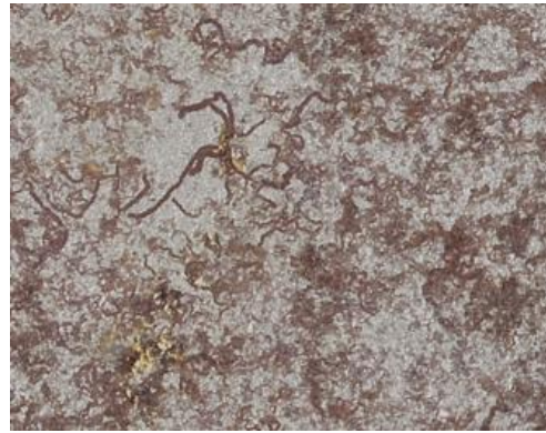
Figure 175 Zoomed areas of CS3B showing a mix of filiform and general corrosion
