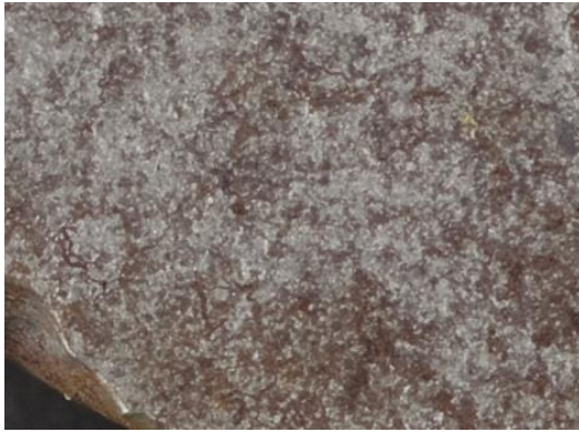
Figure 174 Zoomed area of CS3B showing the effect of surface profile on the corrosion pattern
