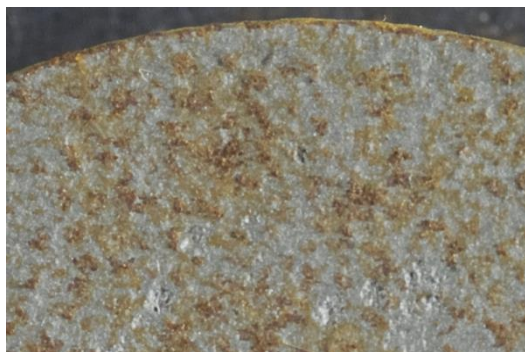
Figure 208 Zoomed area of S10CS5A displaying mainly yellow-brown corrosion
