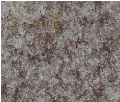
Figure 184 Zoomed area of corrosion on PC1A showing filiform corrosion and a small area of light coloured general corrosion
