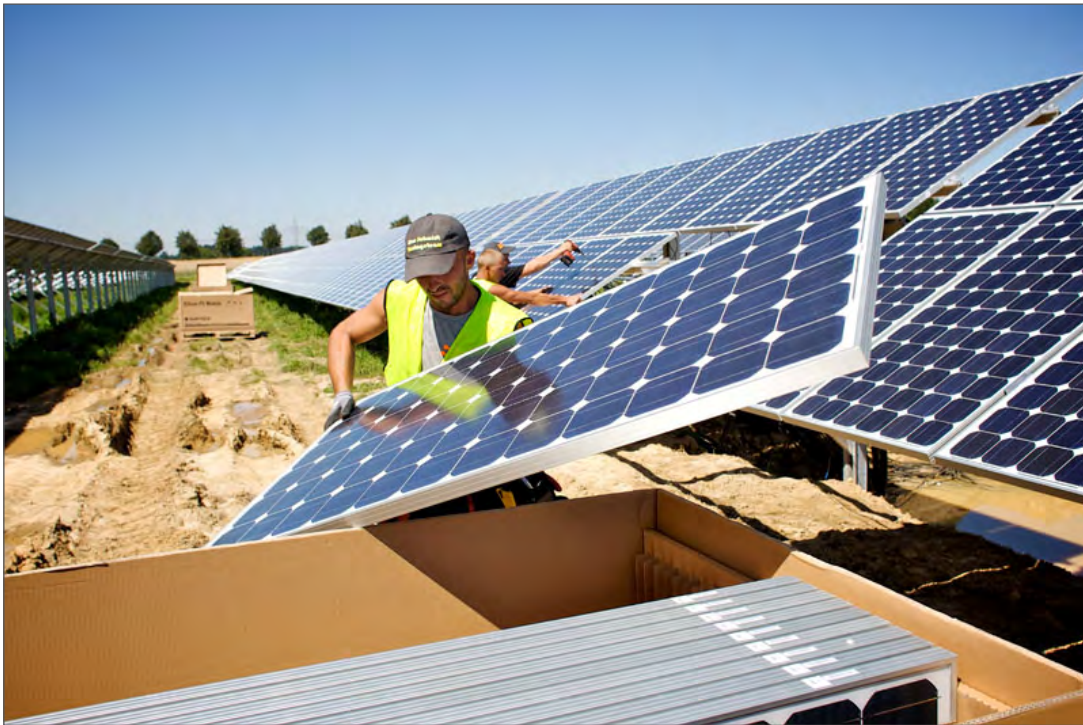
Construction of the ground-mounting photovoltaic system in Altötting/Oberkastl, Bavaria, Germany, July 2009. Photo: Windwärts Energie GmbH / Photographer: Mark Mühlhaus/attenzione (CC BY-NC-ND 2.0)
