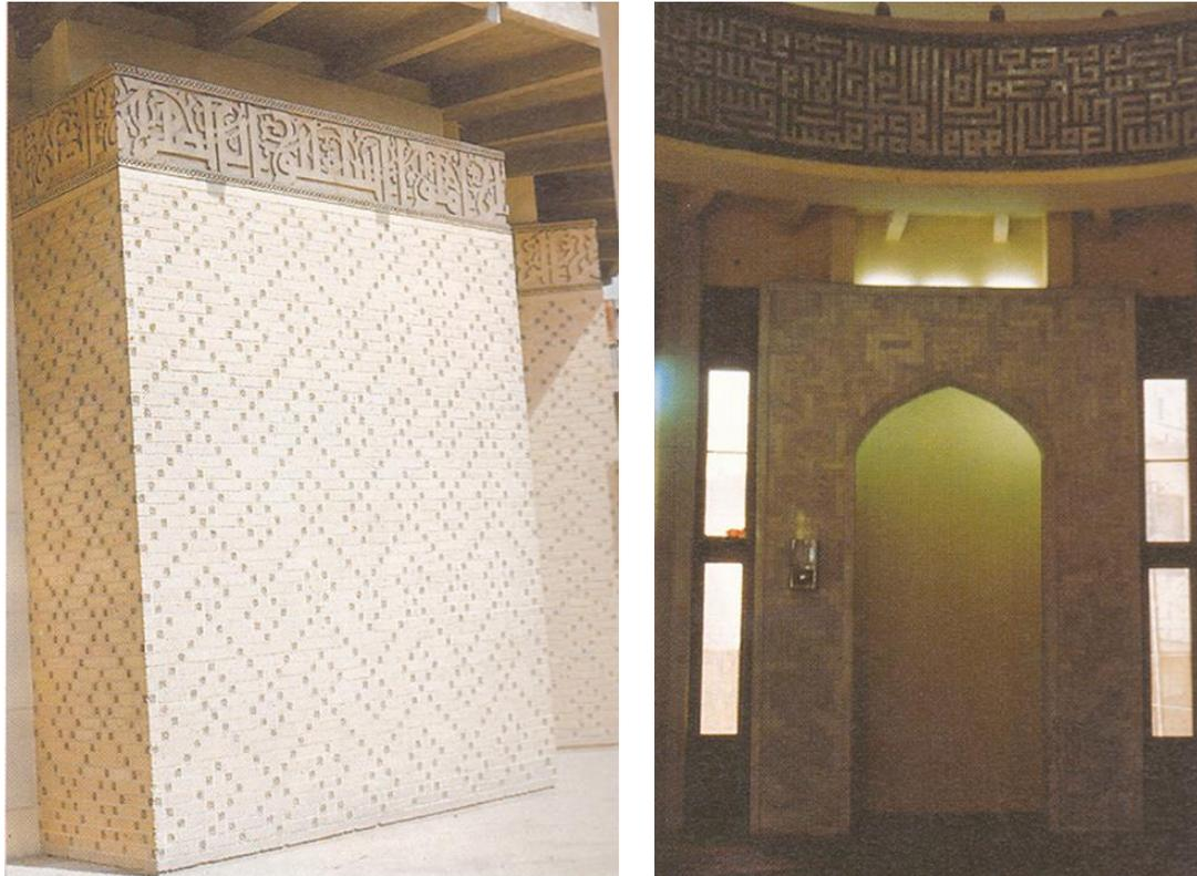
Figure 8.5: Left: prayer hall details of the three-dimensional wall that supports the dome. Right: mihrab concave unit. Source: (Kanan, 1990, p. 46).
