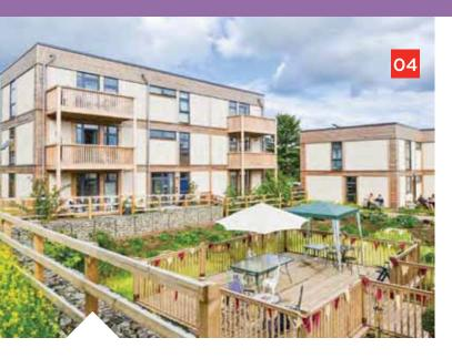
The completed LILAC project, made from straw-based panels assembled at a flying factory nearby, with rainwater harvesting and SUDs at its heart. www.lilac.coop
