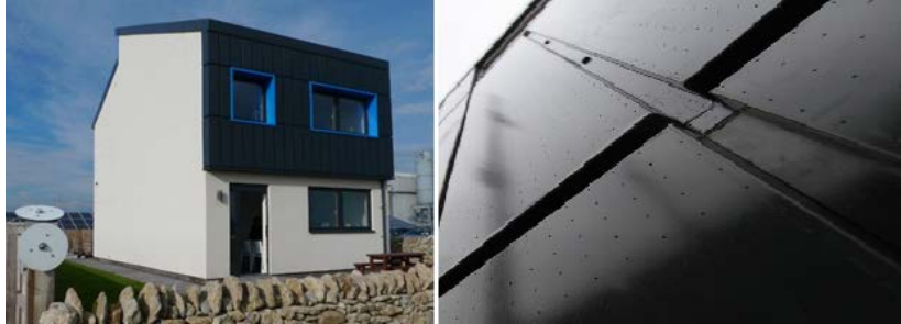
Figure 1 Solcer House, Bridgend, Wales (latitude 52^{\circ} ). Left: The TSC is located across the external area of the upper floor (dark grey/black). Right: Detail of the metal cladding/perforation
