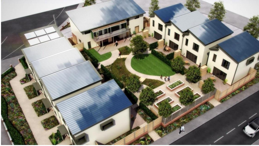
Figure 2-37: The Greenwatt development (Energy Saving Trust 2012)
