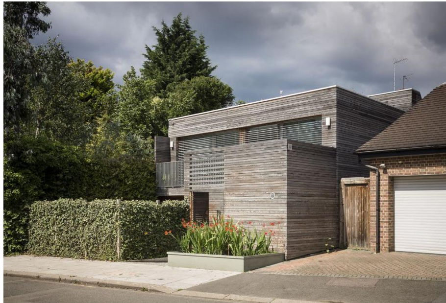
Figure 2-38: The Camden Passive House in London (Ridley et al. 2013)
