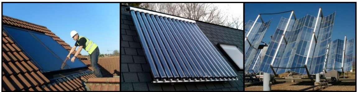
Figure 2-23: Solar thermal energy systems: flat panels (left), evacuated tubes (centre), and parabolic collectors (right) (Weiss 2003)
