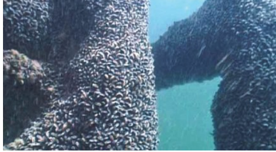
Figure 1.11: Fouling generated on the foundation of an offshore wind turbine.
