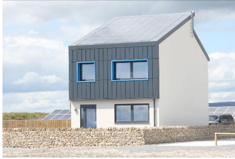
Figure 1. SOLCER House featuring its PV roof and 1 st floor transpired solar air collector (TSC)
