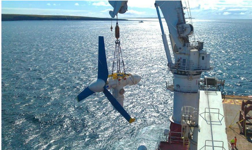
Figure 2.15 Installation of the AR1000 tidal turbine Source: Jupiter Hydro Inc., 2012
