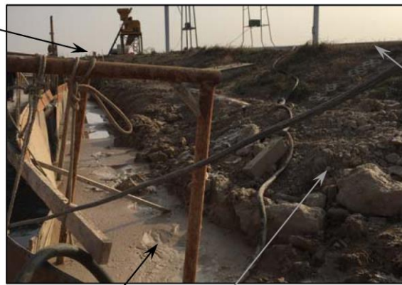
Slurry trench
