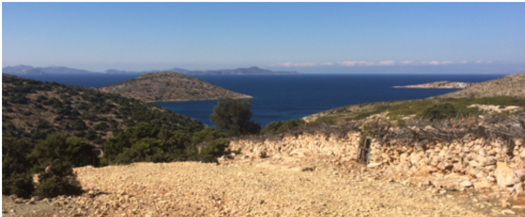
Figure 173 - The road/path to Vroulia is unsurfaced. During the heavy winter rains, both sediment and stones are washed down the path. The water cuts grooves into the surface, restricting vehicle access and flushing further sediment into the bay.
