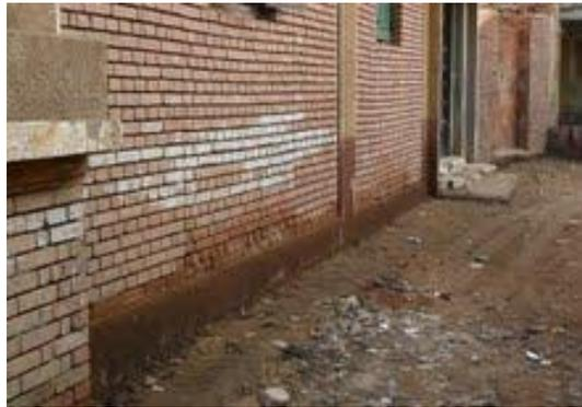
Figure 1.4: Effect of groundwater on the foundations of buildings
