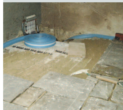
St Fagans Castle. Electric under-floor heating was introduced into the kitchen, the flagstone floor acting as a heat reservoir.
