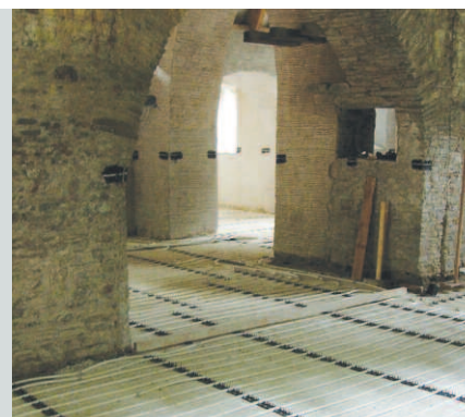
St Teilo's church: Under-floor pipework being laid inside the church on top of a limecrete base. The flagstone floor acts as a heat reservoir and the system is controlled by hydrostats located in the roof-space.
