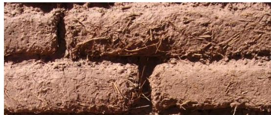
Figure 2-2. Composite mud and straw bricks [13].
