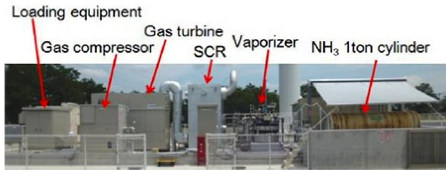
Fig. 25. Photo of the experimental facility of \text{NH}_3 -air and \text{NH}_3 - \text{CH}_4 -air combustion gas turbine power generation [222]. Courtesy of NH3 fuel association.
