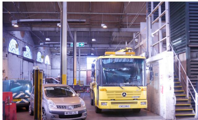
Interior has been in use as a vehicle maintenance shed for over a century
