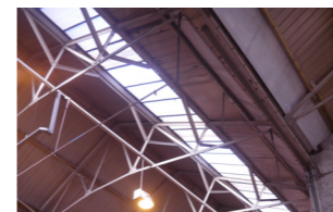
Clean, repair and decorate trusses and structure
