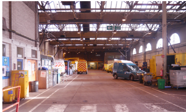
The building has a spectacular daylight, open space
