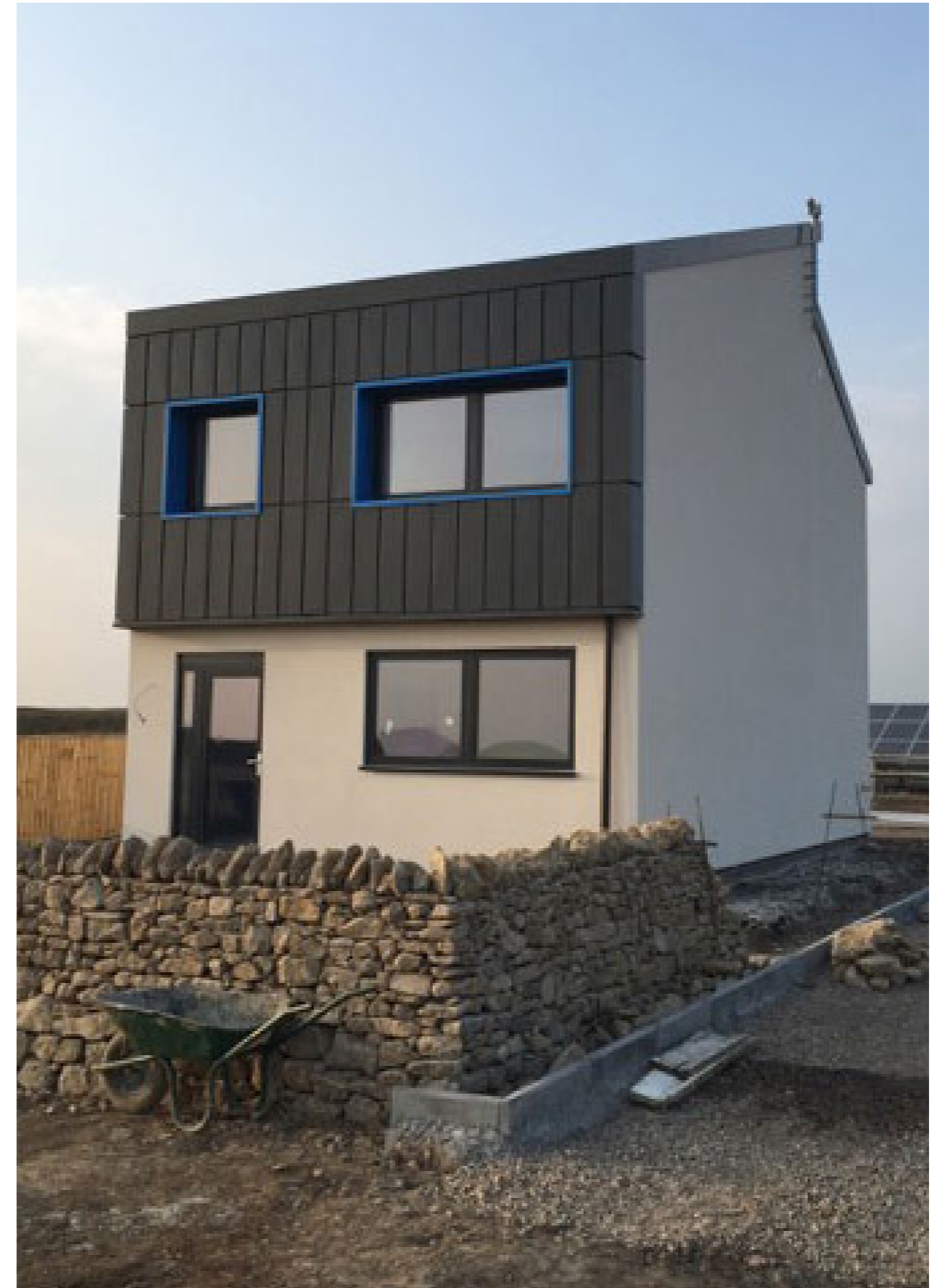
Solcer House, incorporating Transpired Solar Collectors from http://www.cardiff.ac.uk/archi/news-items/solcer-house
