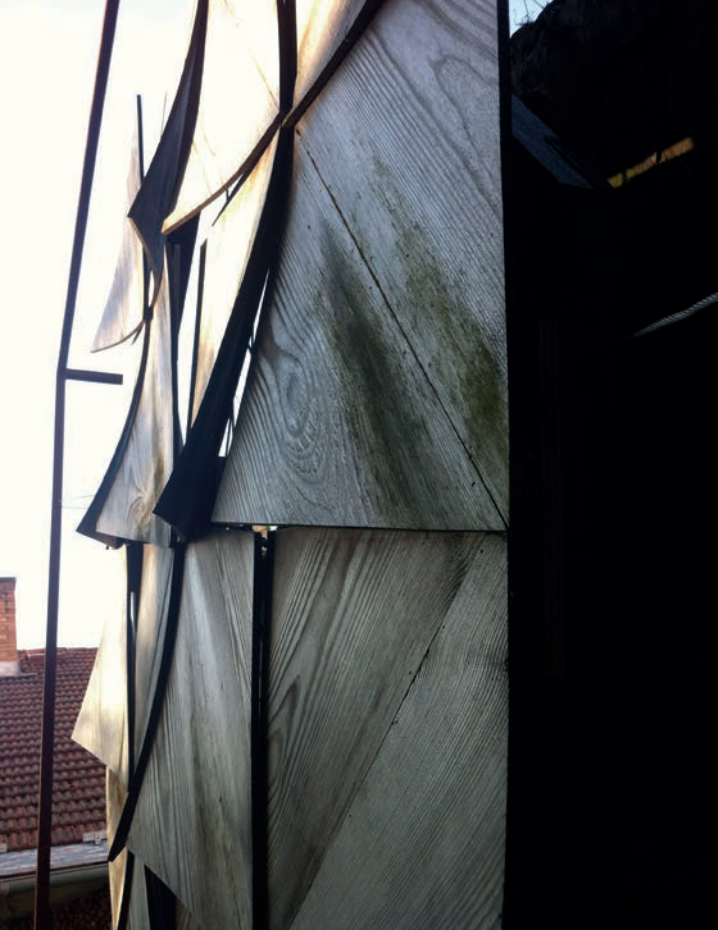
Figure 11: Ray 2 Prototype after Three Years of Being Exposed to Weather and Biotic Conditions (photo: Yildirim 2016)
