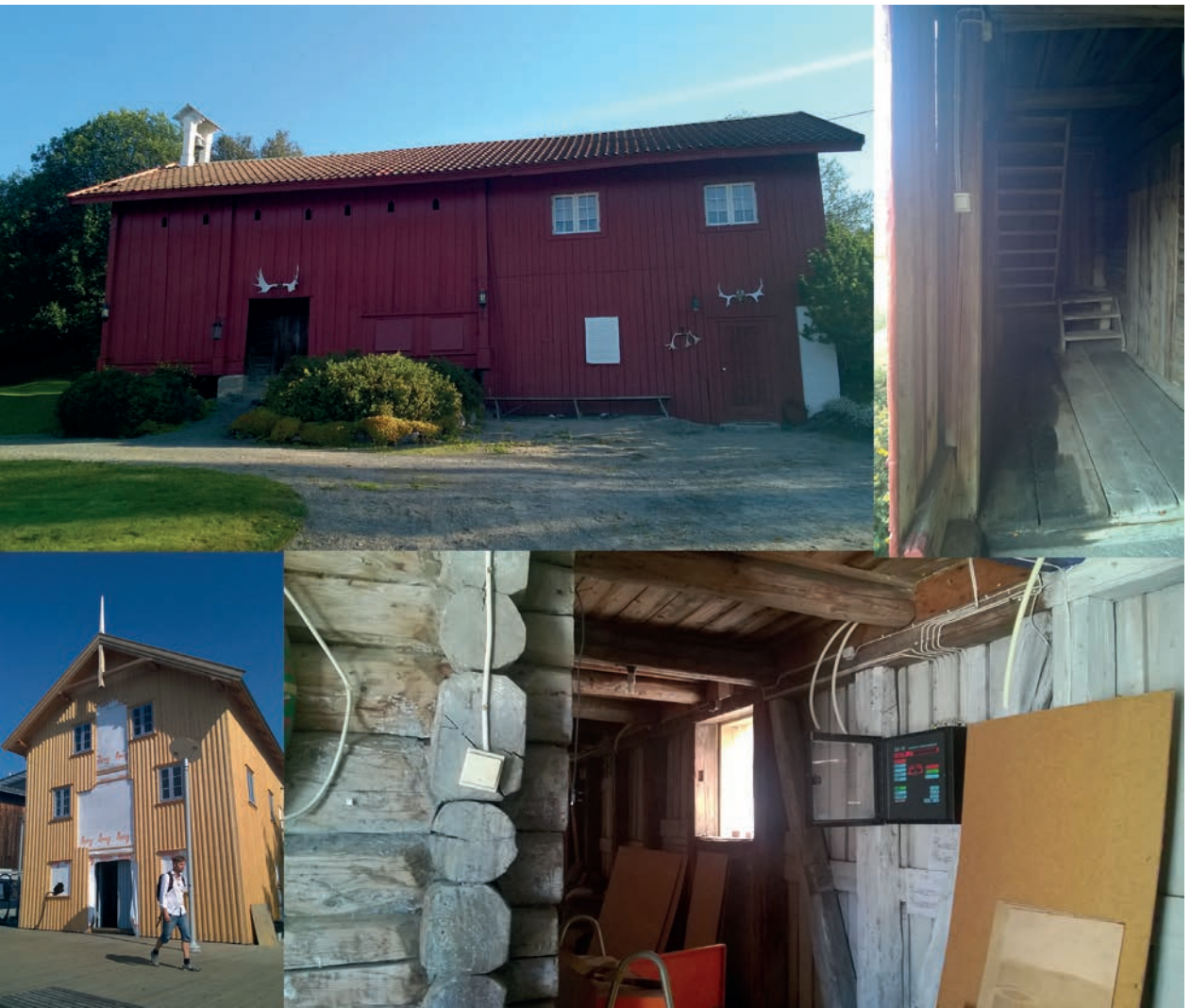
Figure 71: The Unclimatized Spaces, so called Onion System, in Norwegian Traditional Architecture (photo: Davidová 2015)
