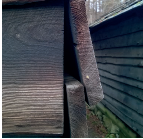
Figure 4: Panelling of Storehouse from Nes, Øvre Valdsaroy in the Open-Air Museum in Oslo (photo: Davidová 2016)
