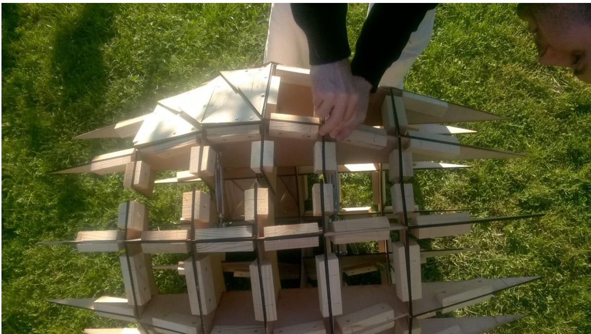
Figure 9: The Waffle Structure with on Place Improvised Wooden Slats to Fix the Panels (Photo: Prokop 2017)
