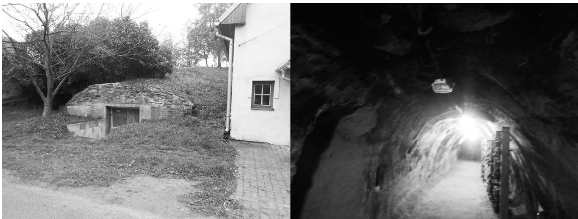
Figure 1: a/left: Combination of Subtractive and Additive Technique on Traditional Wine Cellar in Znojmo, South Moravia, Czechia – these generate constant climate for white wine fermentation about 7-15°C (photo: Davidová 2014) b/ right: Traditional Wine Cellar in Znojmo, South Moravia, Czechia Largely inhabited by Algae - according to the wine grower the algae helps to generate the targeted climate and algaeless cellars don't perform well (photo: Davidová 2014)
