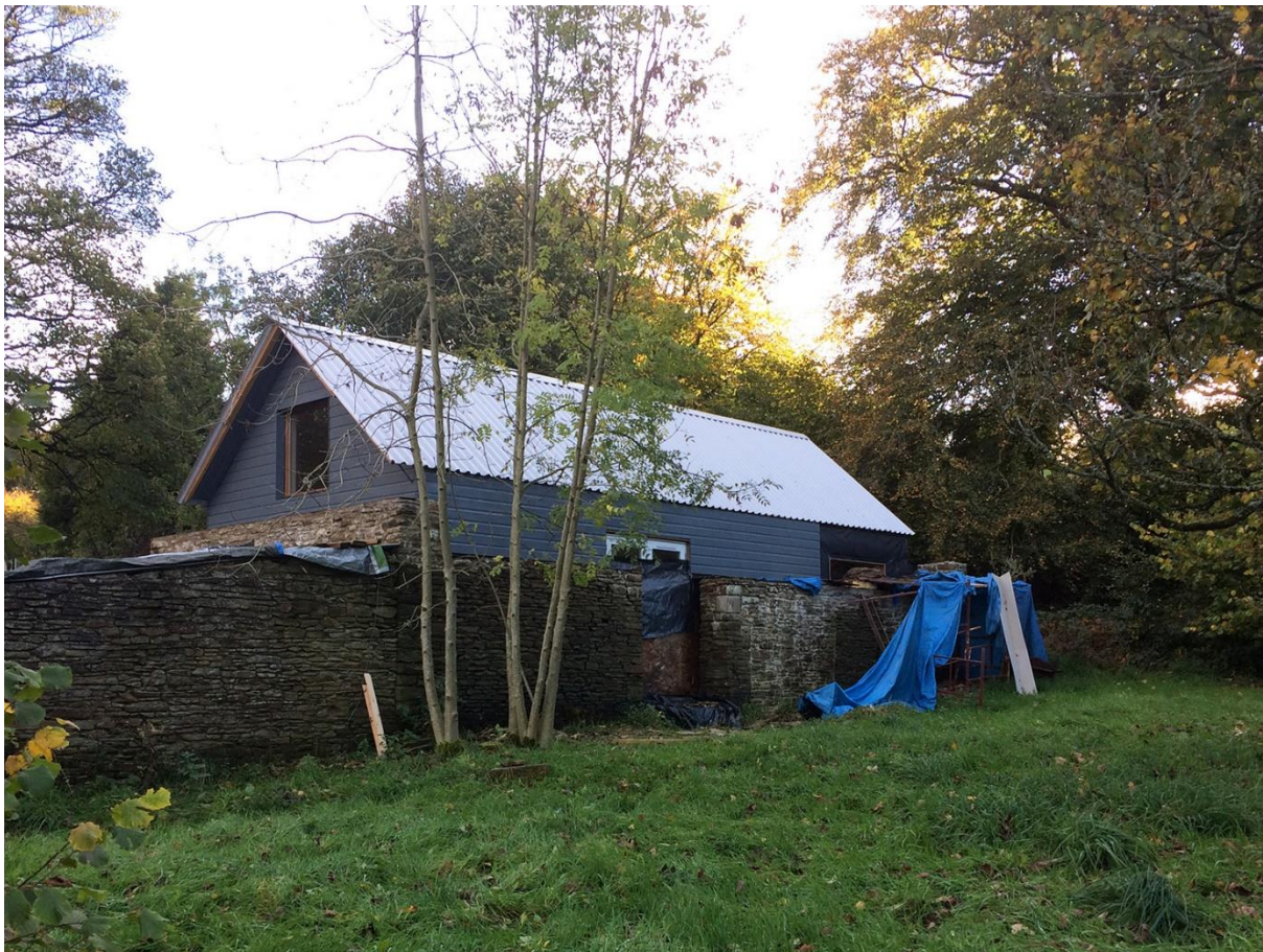
Figure 5.X: The predominantly complete external envelope, awaiting pointing of historic stonework.
