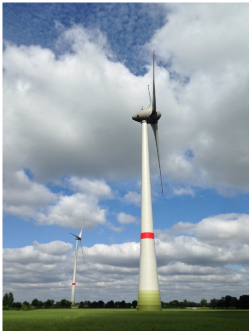
Figure 29a. Onshore wind farm near Diepholz, Germany, with the currently world's highest performing onshore wind turbine, i.e. the Enercon-126, with a hub height of 135m (443 ft), rotor diameter of 126m (413 ft) (Photo: Olaf Schroth 2015)
